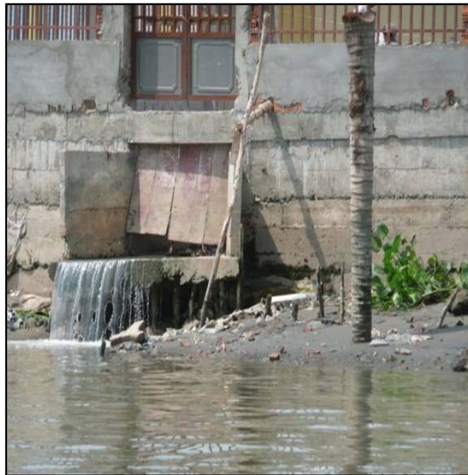
One of the manholes of the Tra Noc Industrial Parks discharges wastewater into Hau River (Photo by S. Benedikter 2009)
