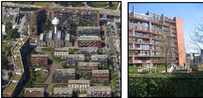
Figure 2. GWL-Terrein, Amsterdam, The Netherlands. Interior green spaces.
