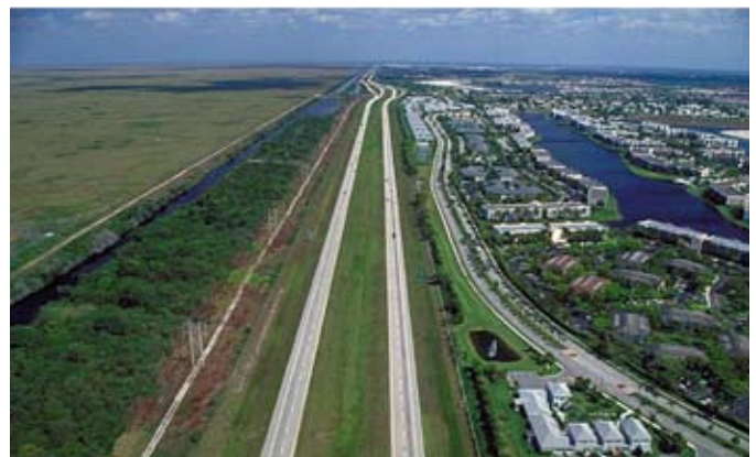
Highways run on top of huge levees separating South Florida urbanization from the Everglades. Image courtesy Pete Rhoads and the South Florida Water Management District.
