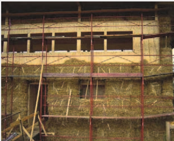
Demonstration building S-House (Source: GrAT)
