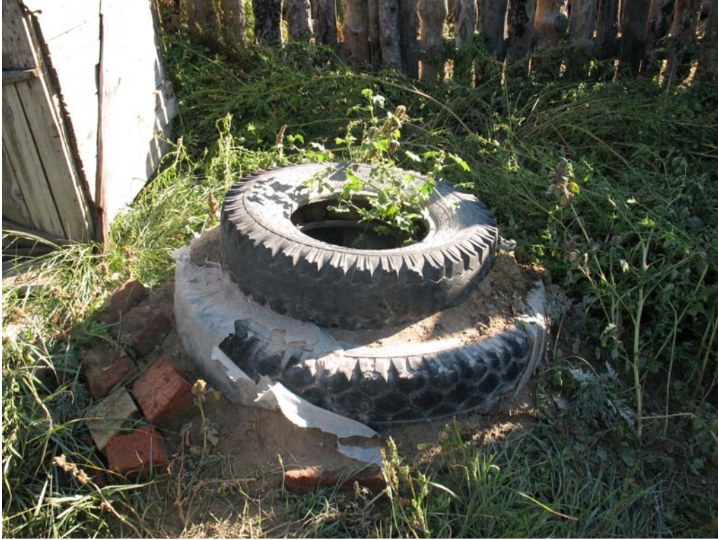
Photo 7: Special hole for greywater discharge
