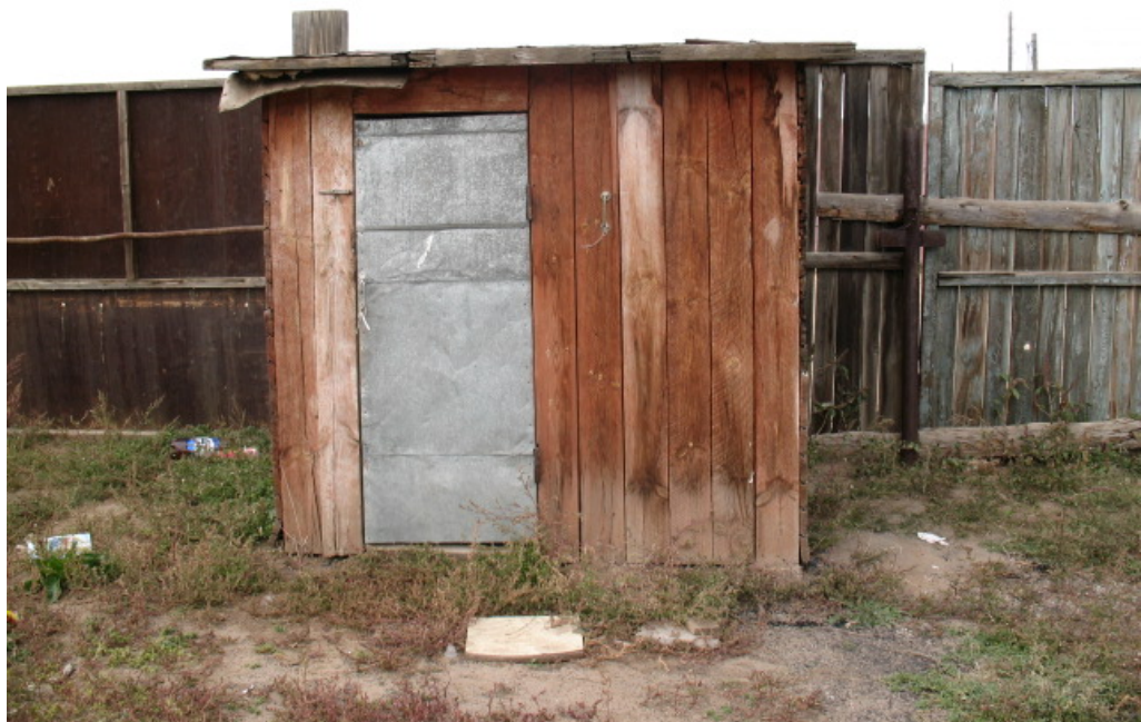
Photo 8: Pit latrine (outside view)
