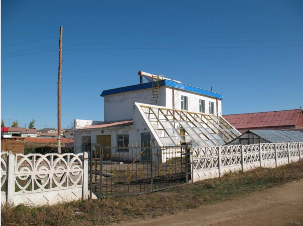
Photo 2: Public bathhouse (back side)
