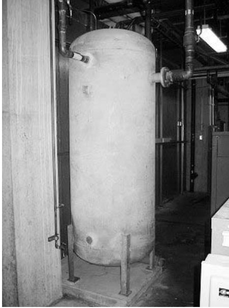
Figure A.9: Vertically oriented tank
