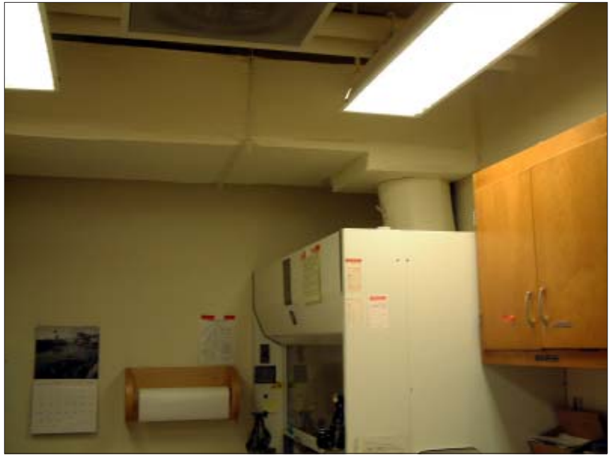
fume hood vent
