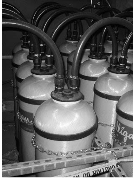
Figure A.10: Multiple tanks
