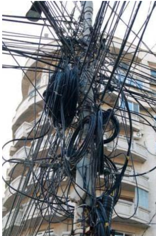
Figure 4-6 Cable Jungle in Romania Source: hotnews Romania
