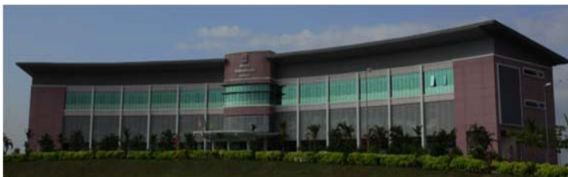
Figure 6 Sepang Municipal Council building
