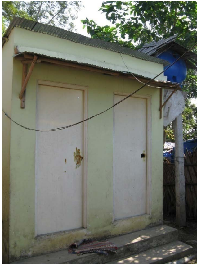
Picture 4: Septic tank latrine and bathroom
