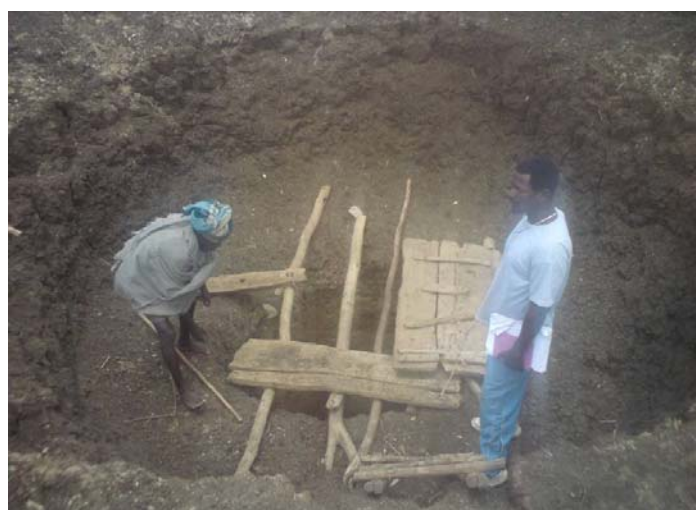
Figure 5: Construction of a V-shaped well
