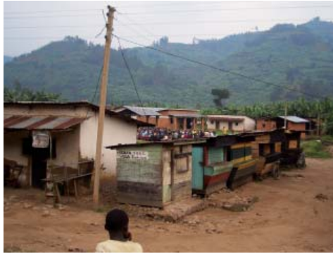
Electricity Grid at Nyamyotsi [NIC]
