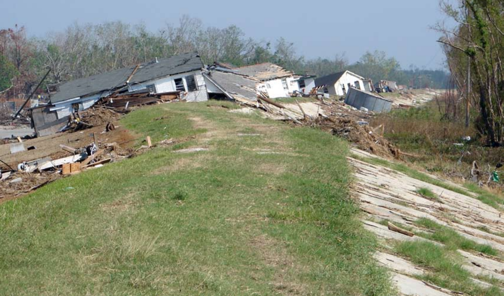
Hurricane Katrina illustrated the dangers of living below sea level. Photo courtesy of Ray Seed.
