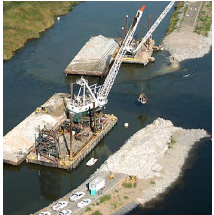
Levee breaches can take weeks or months to repair. Photo courtesy of Ray Seel.
