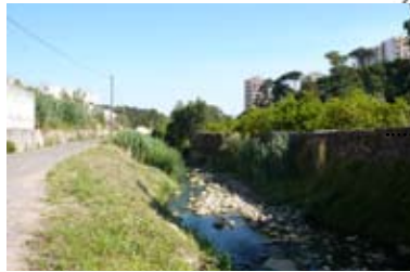
Existing Abandoned Road
