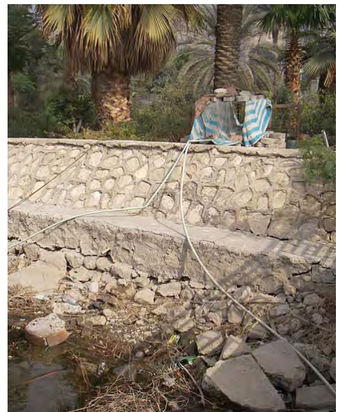
FIGURE 113. Unused vegetated terraces in Maadi
