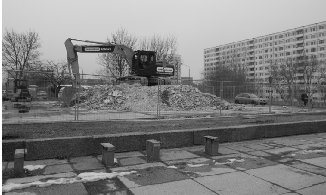
Figure 3.4.6: Housing demolition in a prefab housing estate
