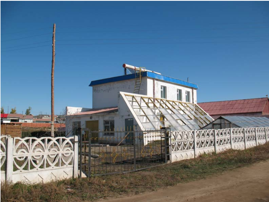
Photo 2: Public bathhouse (back side)
