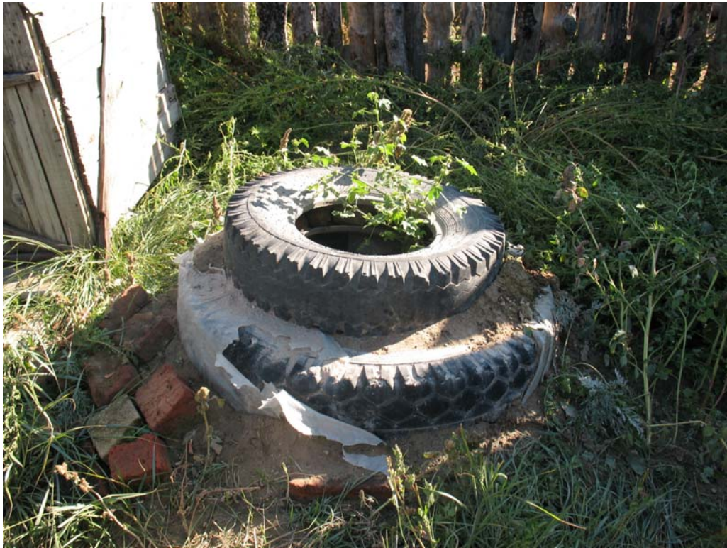
Photo 7: Special hole for greywater discharge
