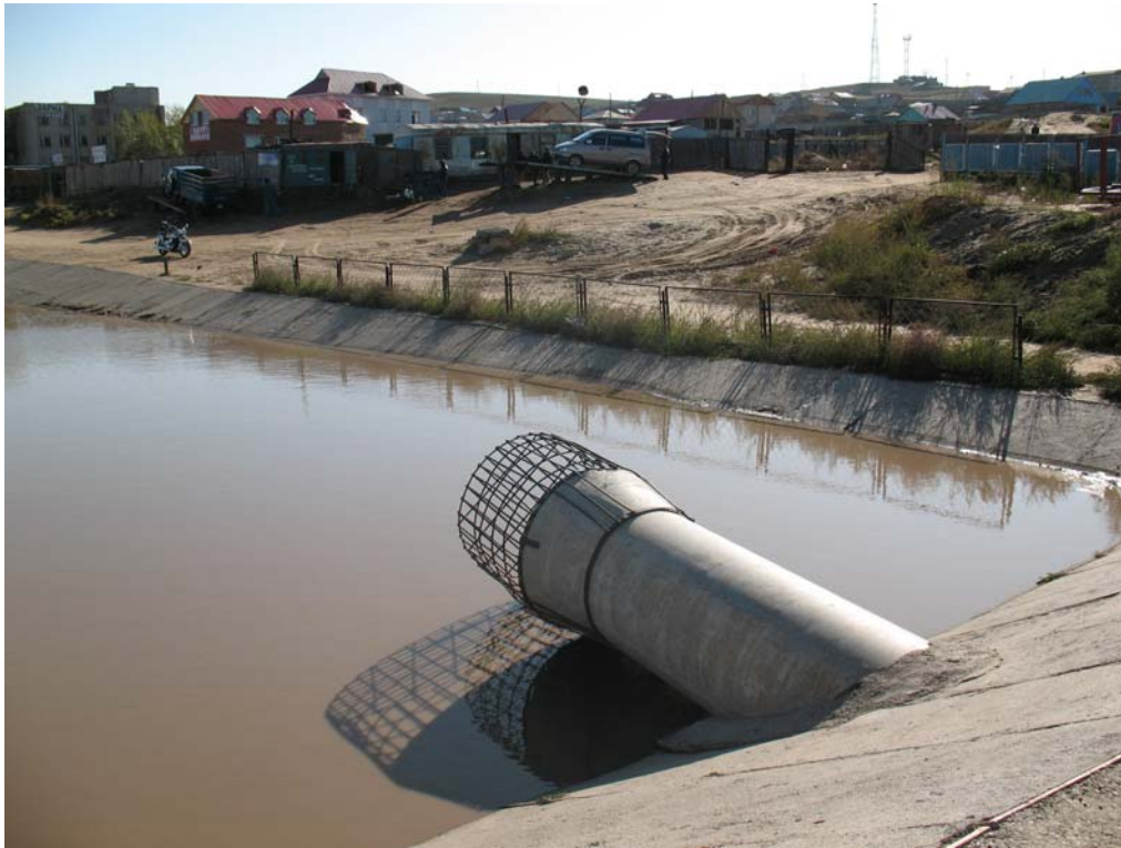
Photo 9: Stormwater storage basin
