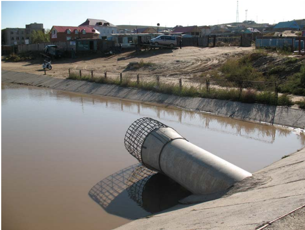
Photo 9: Stormwater storage basin
