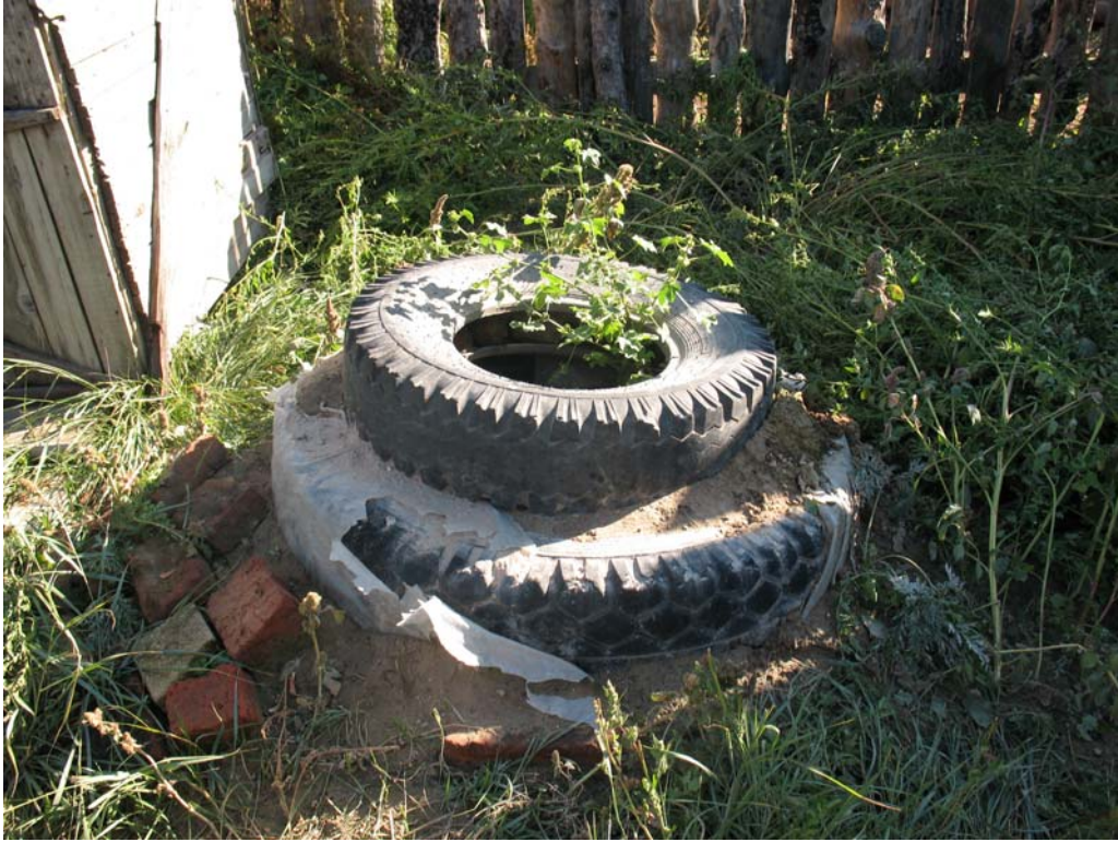
Photo 7: Special hole for greywater discharge
