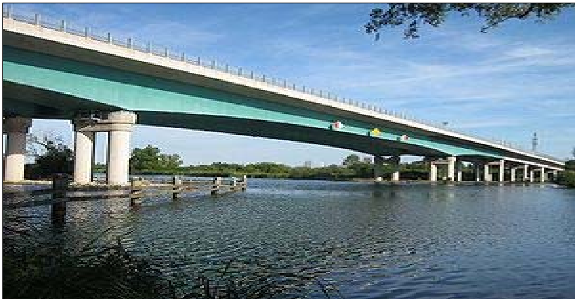
Figure 4: Bridge over the Peene (A20)
