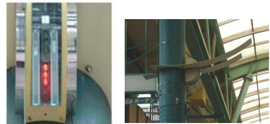
Fig.3 VLC on LED street light
