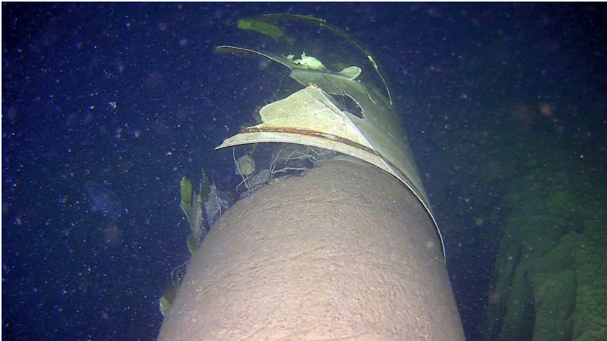
Figure 3 The damaged Balticconnector pipeline (Rajavartiolaitos, 2023)
