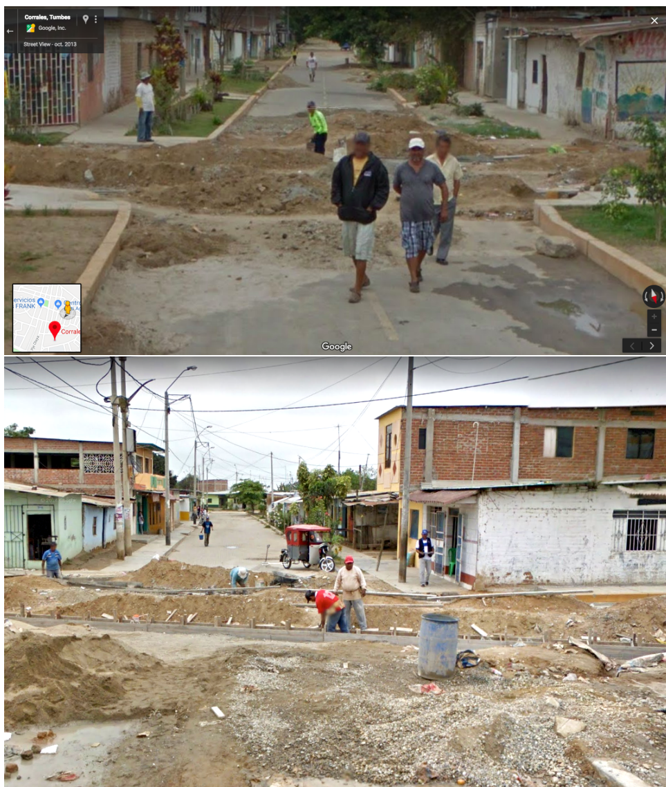
Figure A2 Sewerage project under implementation
