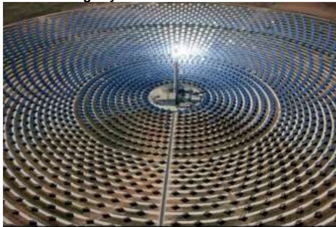
Figure 18: Gemasolar power plant 74 of 20MW with central tower receiver, a heliostat field on 185ha of land and a molten-salt heat storage system
