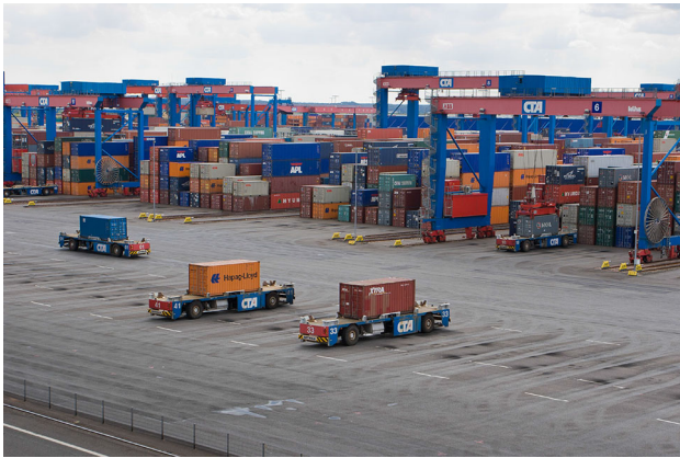
Fig. 1 Gantry cranes at container terminal Altenwerder, Jessen (2020)
