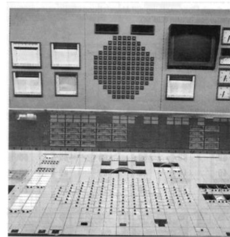
Compatible Placement of Controls, Displays, and Symbols for the Fuel Elements in the Control Room of a Nuclear Power Plant
