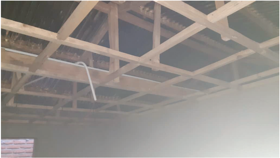
Figure 13: Ceiling structure on hostel houses /Source: Chingalire 2022
