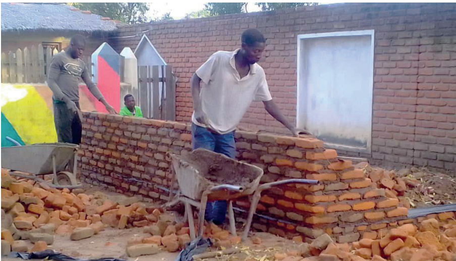
Figure 12: Bricklayer during hostel houses' construction overusing cement / Source: Chingalire 2022
