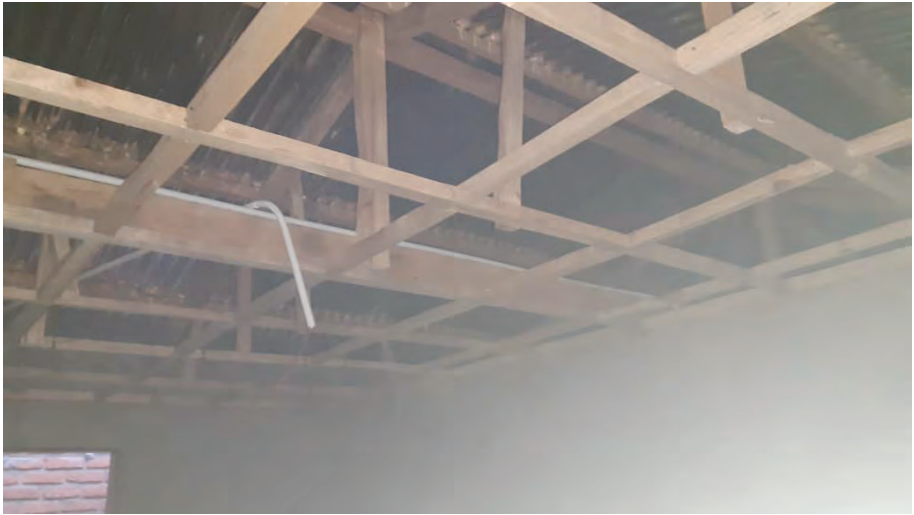
Figure 13: Ceiling structure on hostel houses /Source: Chingalire 2022
