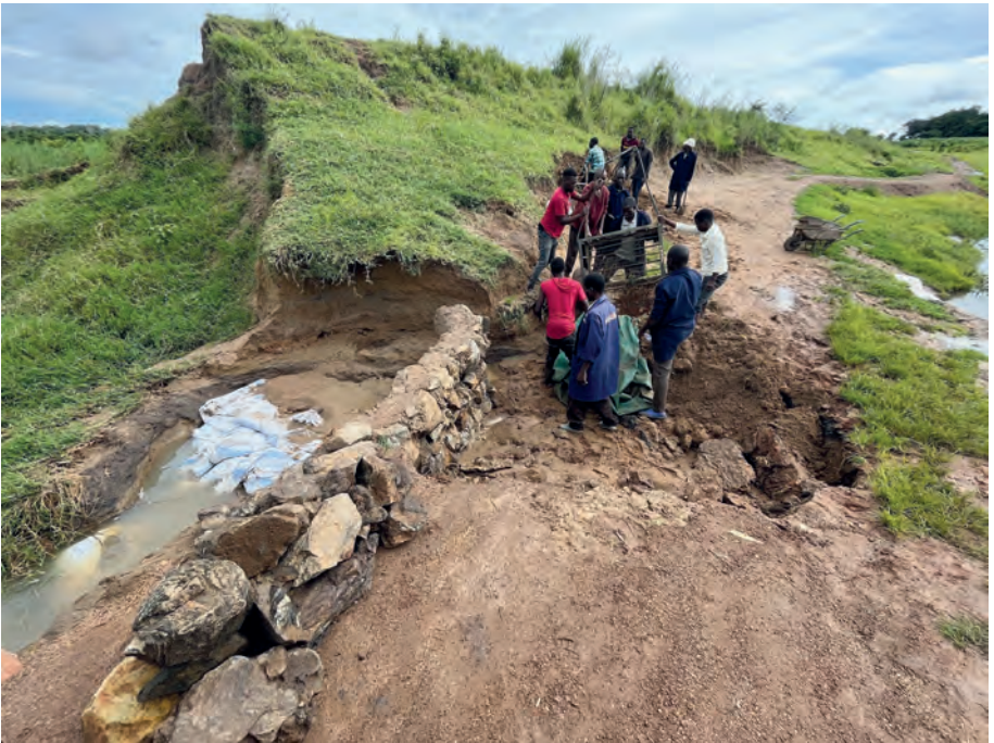
Figure 17: Locals repairing the bridge after the second collapse in February 2023 / Source: Chingalire 2023
