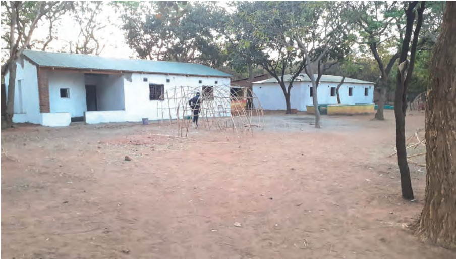
Figure 10: Finalised construction of hostel houses /Source: Chingalire 2022
