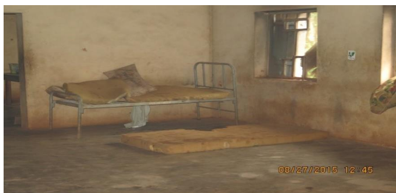
Figure 2. Condition of healthcare centre in the study area
