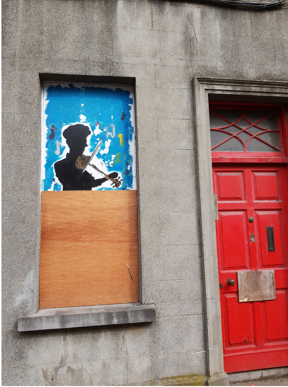
Figure 13.1: Evidence of the efforts to enliven derelict buildings for the Fleadh that have been neglected since. Photograph: Daithí Kearney.
