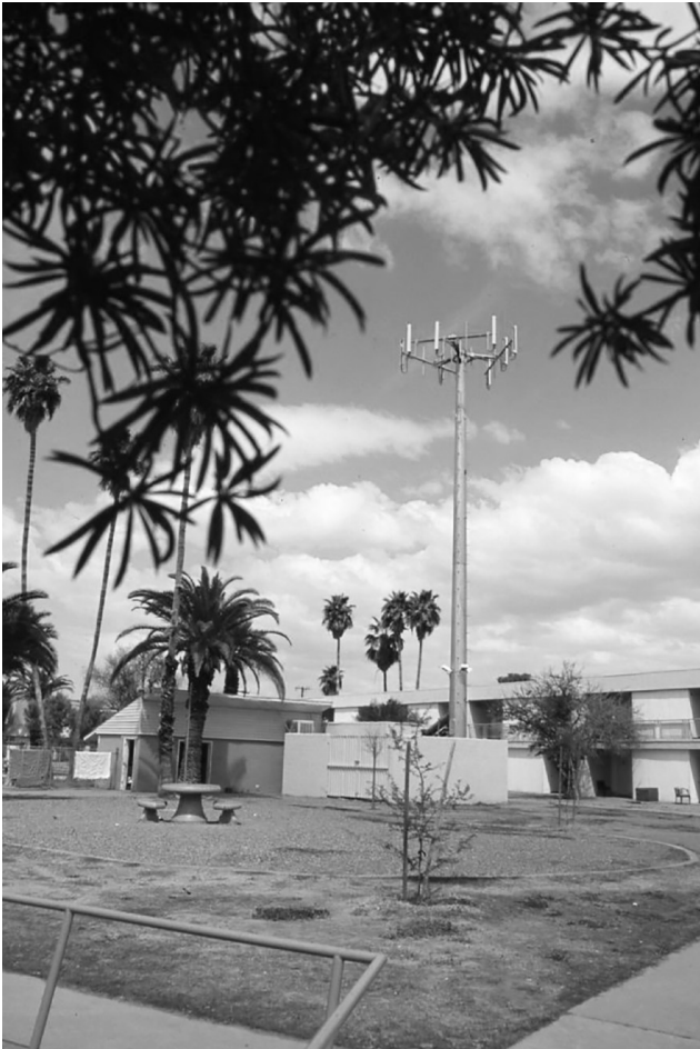
4.1 A typical 2G cell tower. Courtesy of AT&T Archives and History Center.
