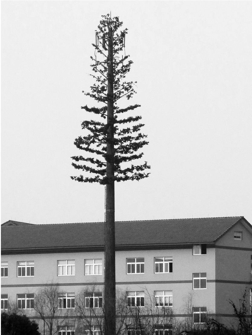
5.4 A disguised cellular mast in the picturesque town of Wuzhen, China. Source: Wikimedia.
