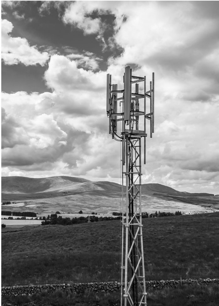
10.1 A 4G cell tower located in rural Scotland, 2018. Courtesy EE.
