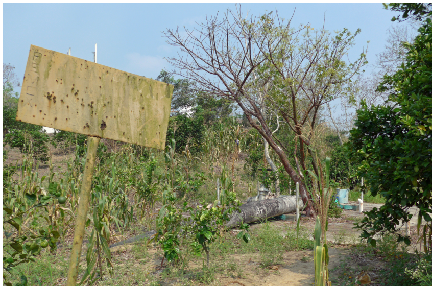
Figure 4.3. Decaying industrial installations—a pipeline and an unreadable sign—amid corn crops and orange trees, Papanthla, Mexico, 2016 © Svenja Schöneich.
