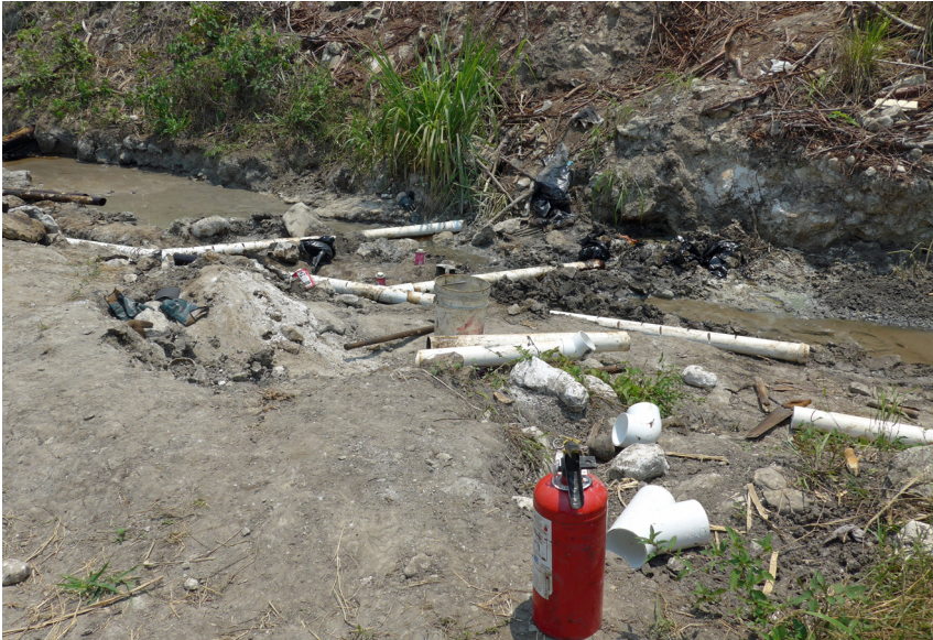
Figure 4.1. A month-old seepage within the river, which awaits repairs, Papantla, Mexico, 2017 © Svenja Schöneich.
