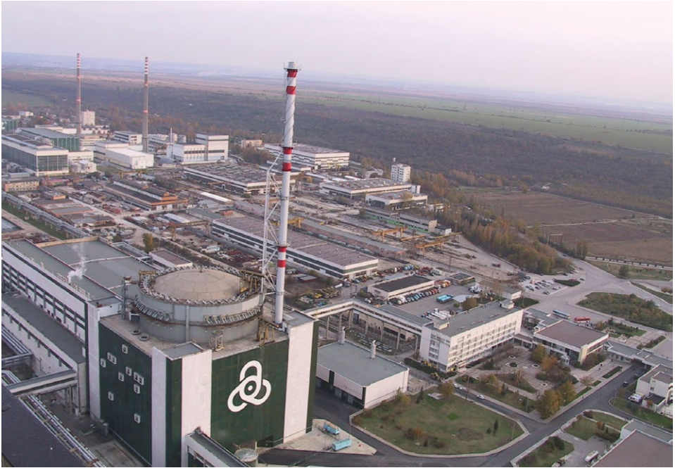
Kozloduy nuclear power plant, Bulgaria. It is being decommissioned through the EBRD-managed Kozloduy International Decommissioning Support Fund (KIDSF). © EBRD
