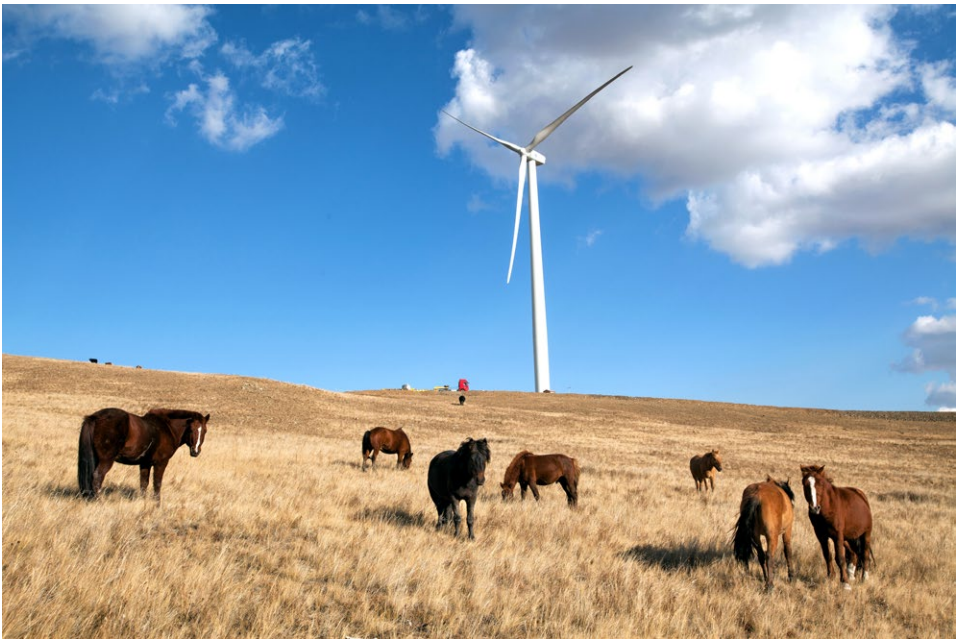
Salkhit wind farm, Mongolia. The first large-scale renewables project in Mongolia and the first new electricity generator in the country for the last 30 years. It was conceived by local investors with early EBRD equity participation. © EBRD
