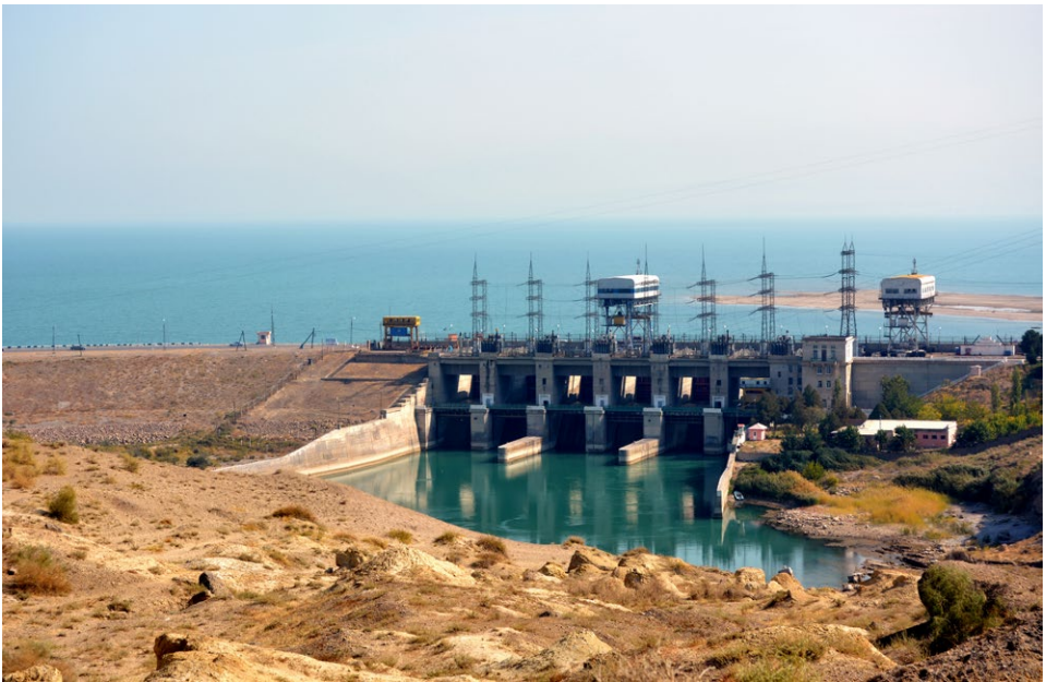
Qairokkum hydropower plant, Tajikistan. The EBRD's support to the rehabilitation of Qairokkum shows how climate resilience can be integrated into an infrastructure investment. © EBRD
