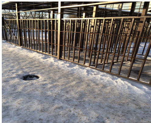
FIGURE 9. Reception facility at an FMS Office in Moscow's Bibirevo district. January 2014. Photo by author.
