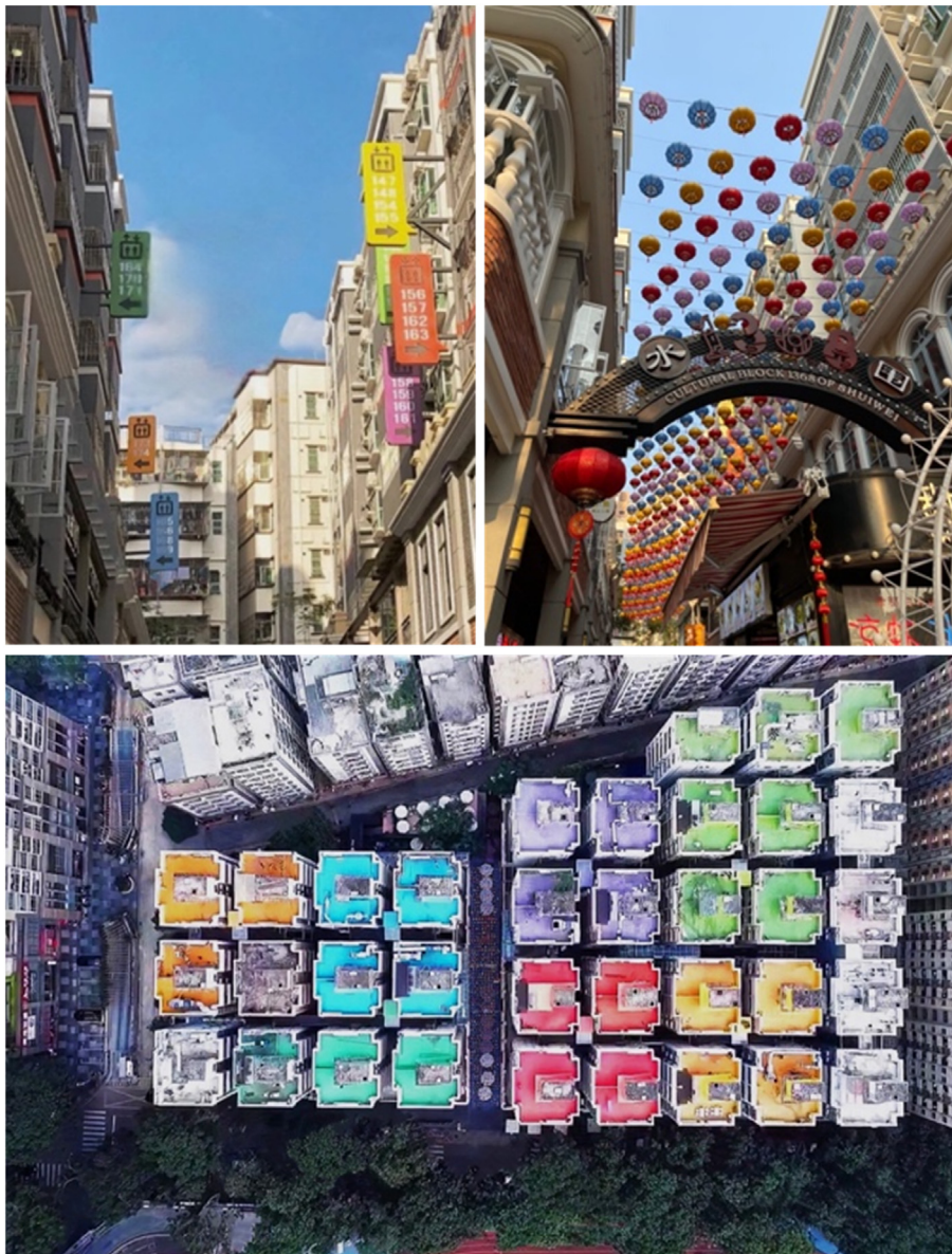
Fig. 4. Residential and commercial environment of Shuiwei after the renovation (photos taken by the first author).
