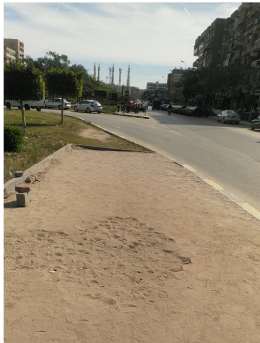
Fig. 3. Showing the now interrupted pavement of the main spine of the neighborhood (Source: the authors).
