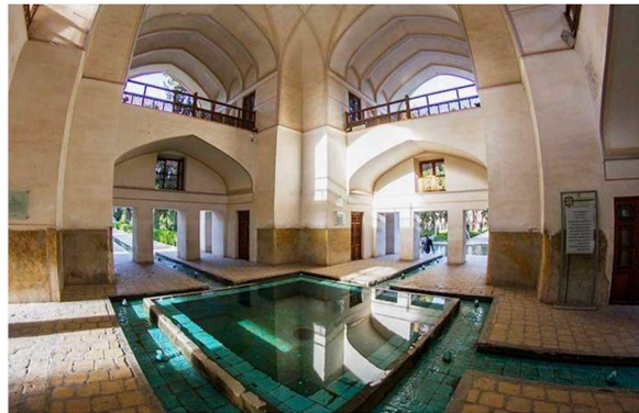
Fig. 4. The kushk in the Fin garden is located at the center of the garden and consists of four vaults (opening) and a dome.
