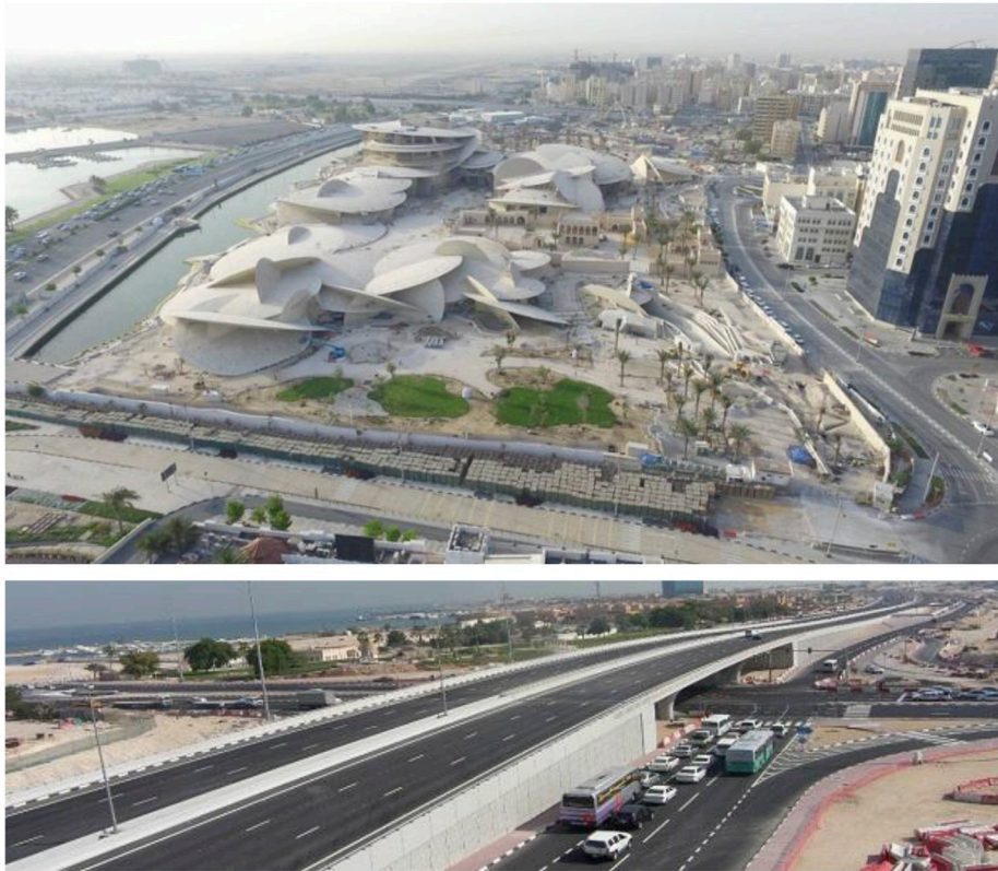
Fig. 18. Aerial views of site access (Source: the Authors).
