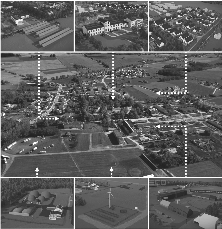
Figure 8.3 Aerial photo 2019 of Lubań and the village revitalization concept, with the Pomeranian Energy Cluster infrastructure designed by Eco-Construction Ltd. (Source: Eco-Construction Ltd). From the top left: (A) solar parking in front of PODR headquarters, (B) renovated mansion house with historical park and the educational path (revitalization finished in 2020), (C) private housing estate. From the lower left: (D) biogas installation, the wind mill turbine, (E) a 40 kW photovoltaic microinstallation and a windmill, (F) the Education and R&D Centre.
