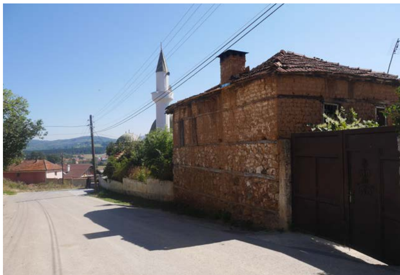
Photo 9: The only old house in the village.
