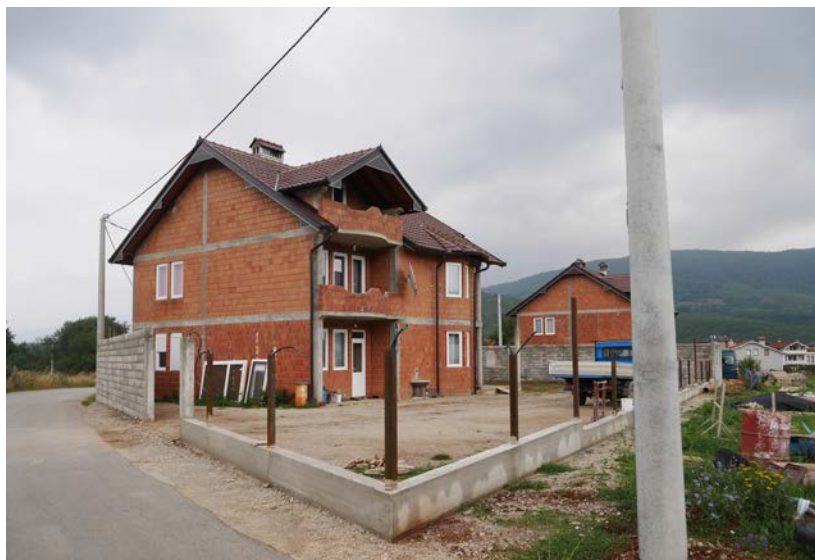
Photo 3: Construction everywhere! New houses under construction in one Opoja village.
