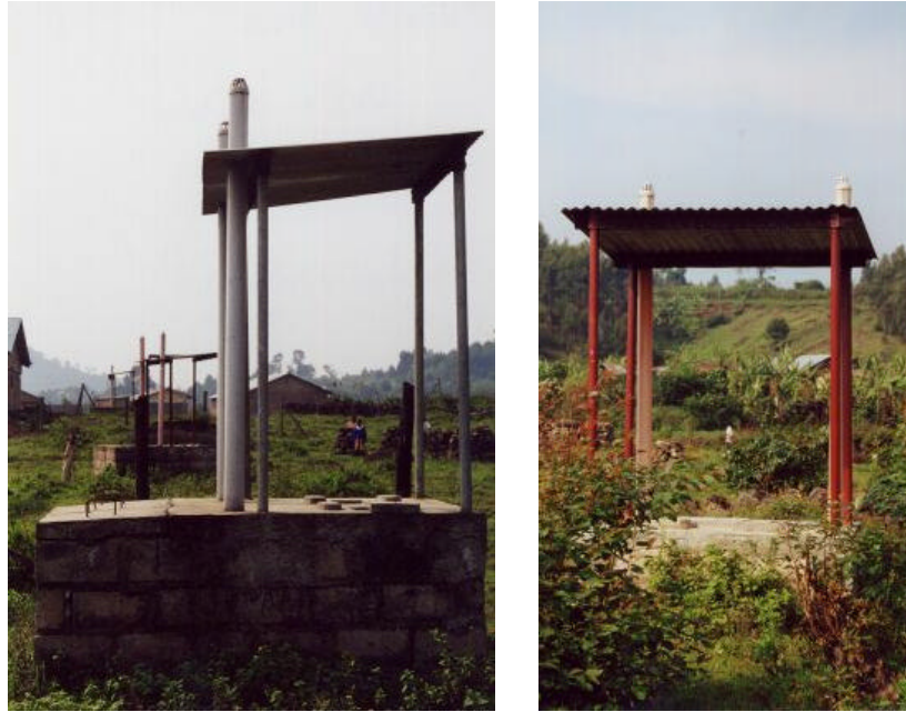
Picture 8: Toilet sub structure.
