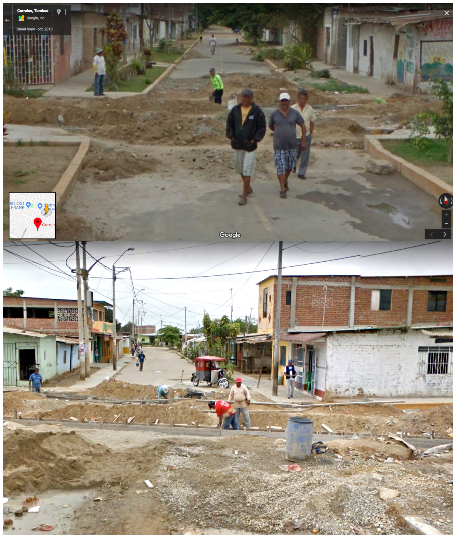
Figure A6 Implemented Sewerage Project with a Completion Rate \leq 60\%
