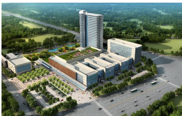
Xiangtan's new flood-resistant hospital, which will follow green building principles and have a trigeneration system for heating, cooling, and power. It will be able to withstand severe weather and flooding through ecosystem-based adaptation measures with large run-off areas and underground storage tanks (photo by Xiangtan PMO/design institute).
