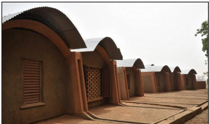
Figure 1: Sustainable housing in Gando, Burkina Faso by Krancis Kere (2011) - uses earth bricks and large roof overhangs for thermal comfort in the houses.
