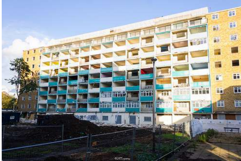
Panel A. Existing building
