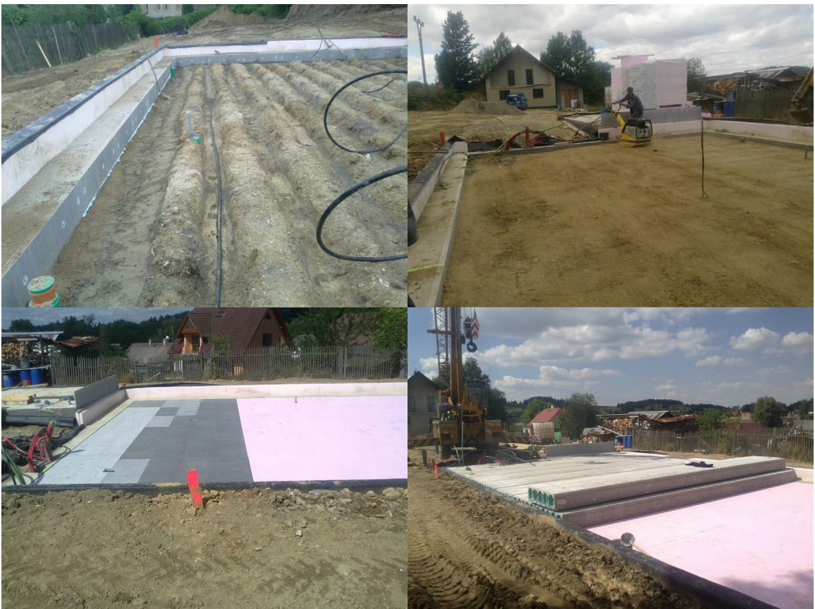
Fig. 2. Realization of low-cost ground storage within foundations.
