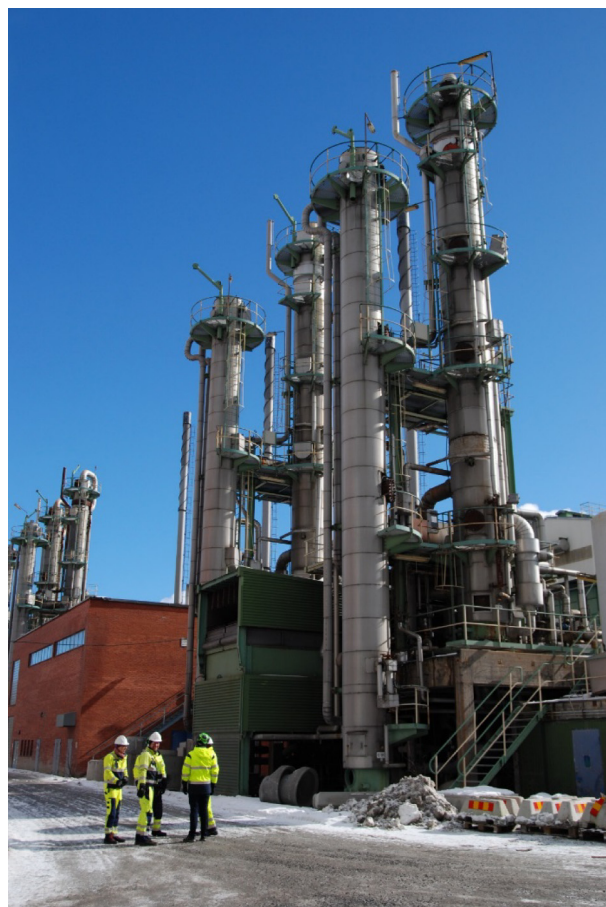
Fig. 1. The four HPC/Benfield CO 2 separation lines at the gas refinery in Stockholm that operated utilizing hot potassium carbonate between 1971 and 2011 (photograph taken 16 March 2018).
