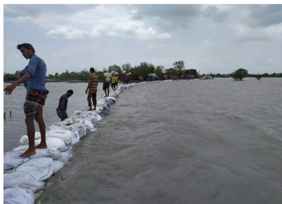
Figure 2(d). Village dweller reconstructed Embankment, Koyra (June, 2020)
