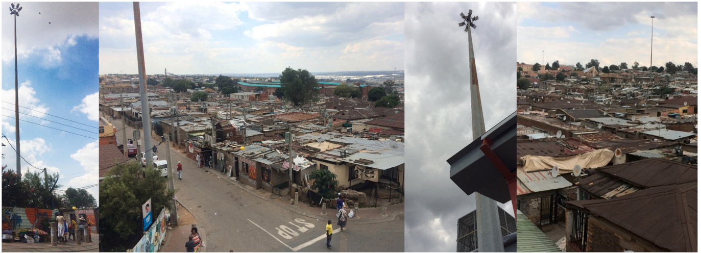
Fig. 1–4. Example of high-mast lighting in Johannesburg, South Africa (David M. Kretzer, 2017).
