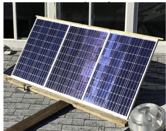
Fig. 3. Three 12 V, 100 W solar panels facing approximate solar noon (1:00 p.m. local time), receive sunlight from 9:00 a.m. to 5:00 p.m.
