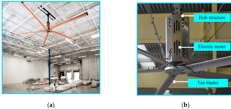
Figure 2. Monstrous fan (a) Physical condition [10] (b) Common structure.
