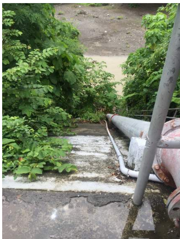
Figure 1B- 21. The 10" pipe connected to the original pump that delivers water to the main canal
