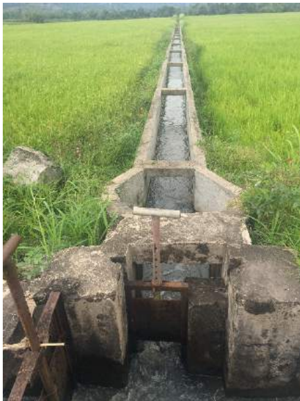
Figure 1A-71. Left: lined; Right: unlined farm ditches
