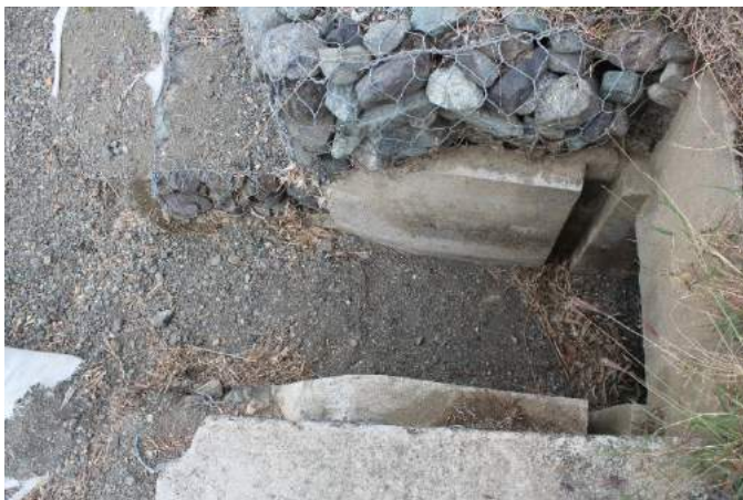
Figure 1A-26. The intake structure with the slots for the wooden gates
