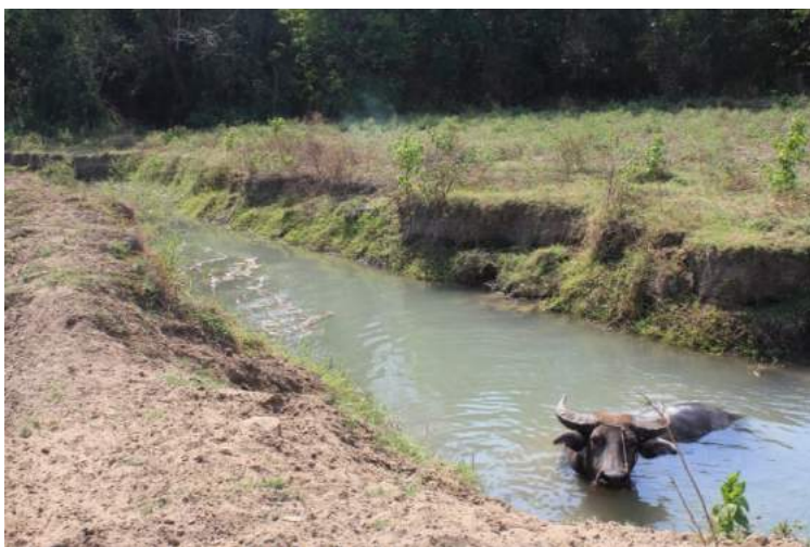
Figure 1A-114. Unlined main canal Source: Author's capture
