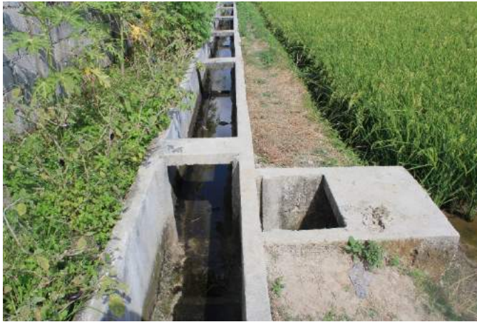
Figure 1A-10. The concrete-lined main canal with a simple turnout gate using slots and wooden slabs as gate
