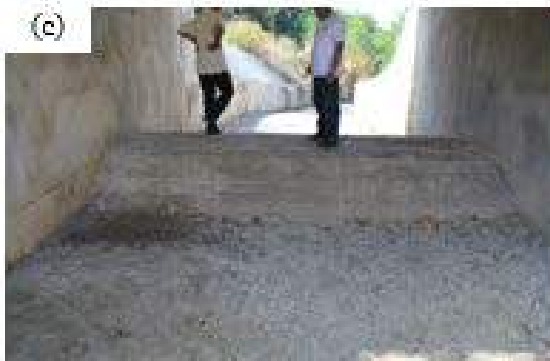
Figure 1A-47. (a) The entranceway to the concrete spillway; (b) the level spillway channel; (c) the hump along the spillway channel to increase storage capacity of the dam; (d) the spillway chute to channel excess water from the dam to a creek
