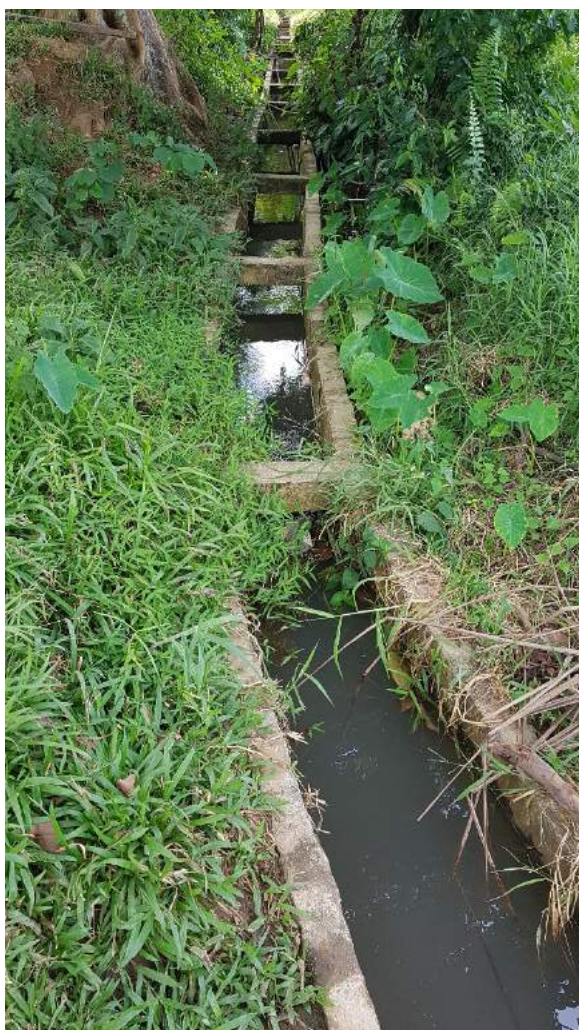
Figure 1C-14. The main canal near the dam and at the end of concrete lining
