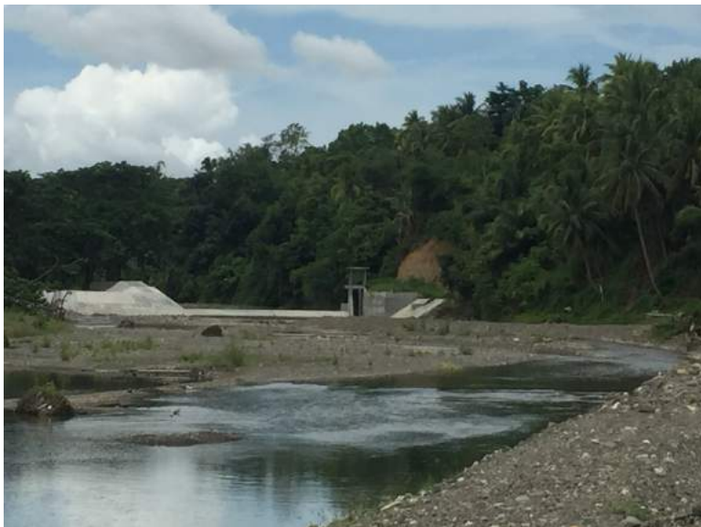
Figure 1B- 16. Construction of the new dam
