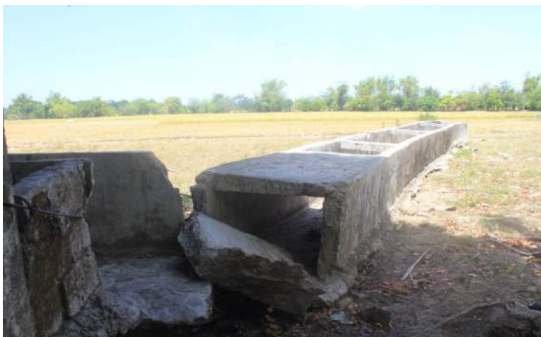
Figure 1A-118. Detached Main canal due to typhoon Glenda
