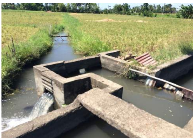
Figure 1A-104. One of the division boxes of the irrigation system with corrugated GI as control gate Source: Author's capture
