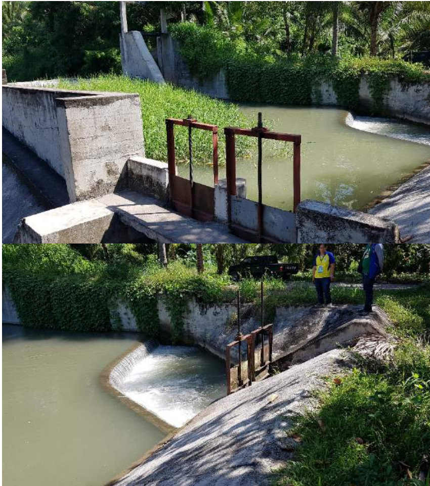
Figure 1C-23. The silt control structure and intake gate
