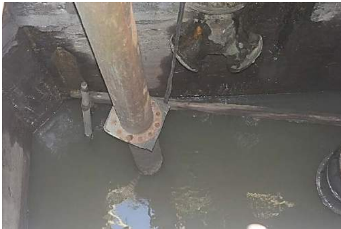
Figure 1A-3. The concrete intake pit for the suction pipes of the Gulap Pump Irrigation System; also shown is the 10-in pipe of the submersible pump
