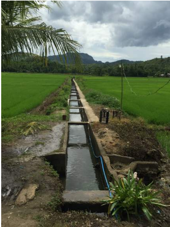
Figure 1B- 32. Main canal of Salcedo CIS
