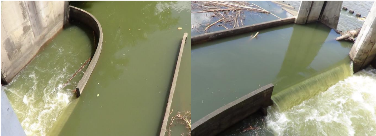
Figure 23. Construction of silt excluder at the MalRIS
