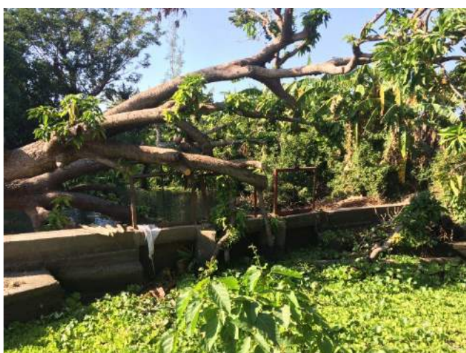
Figure 1A-61. Damaged and non-operational gates due to a tree falling on it during the typhoon Mario in 2014.
