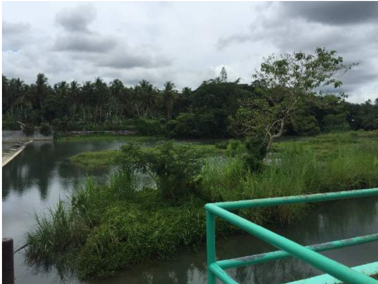
Figure 1B- 15. Dam site showing that dredging is not practiced
