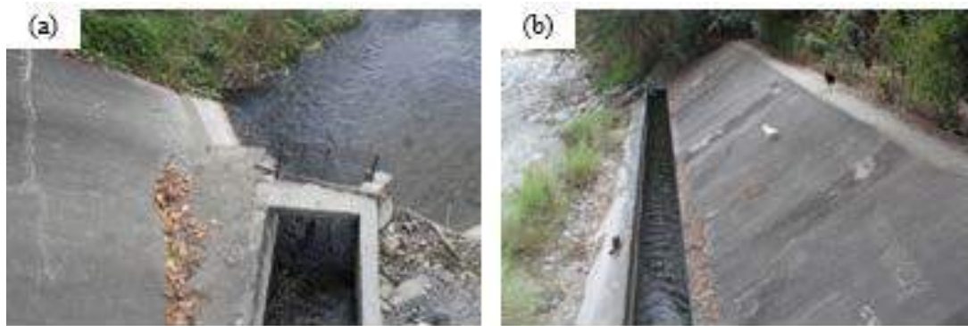
Figure 1A-52. (a) The intake structure with a steel grill to prevent entry of large debris and stones into the main canal; (b) the intake channel at the bottom of the embankment
