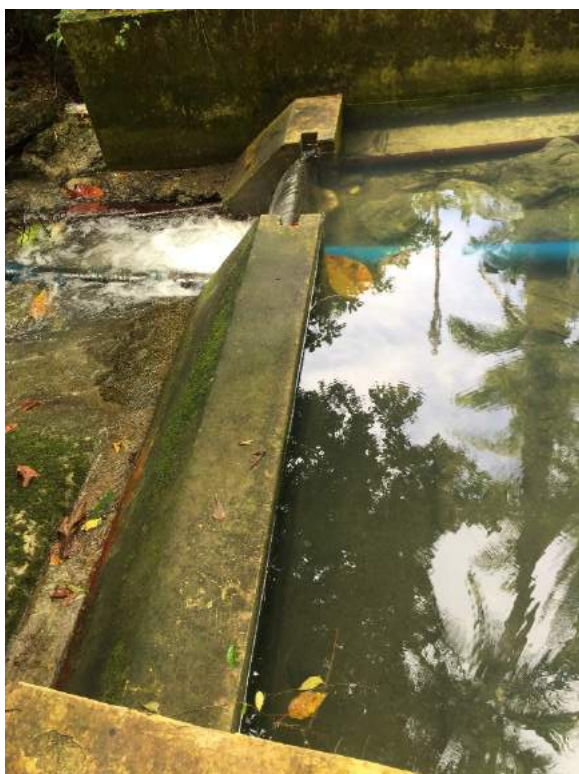
Figure 1B- 8. The diversion dam of the Cambuyo CIP
