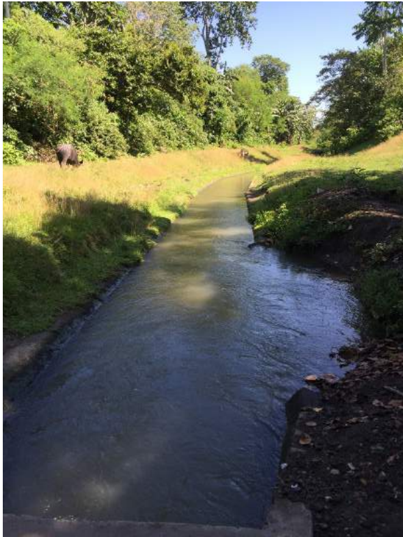
Figure 1C-27. The main canal of Mani CIS from the dam
