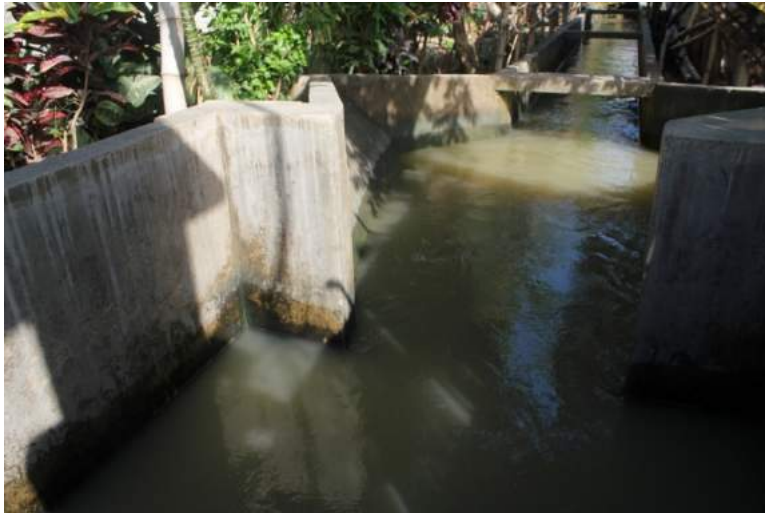
Figure 1A-5. The outlet of the inverted siphon under the road across the concrete sump and pump house; this channels the water into the main canal
