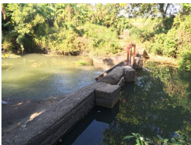
Figure 1A-60. A check gate with one steel gate damaged and replaced with wooden plank
