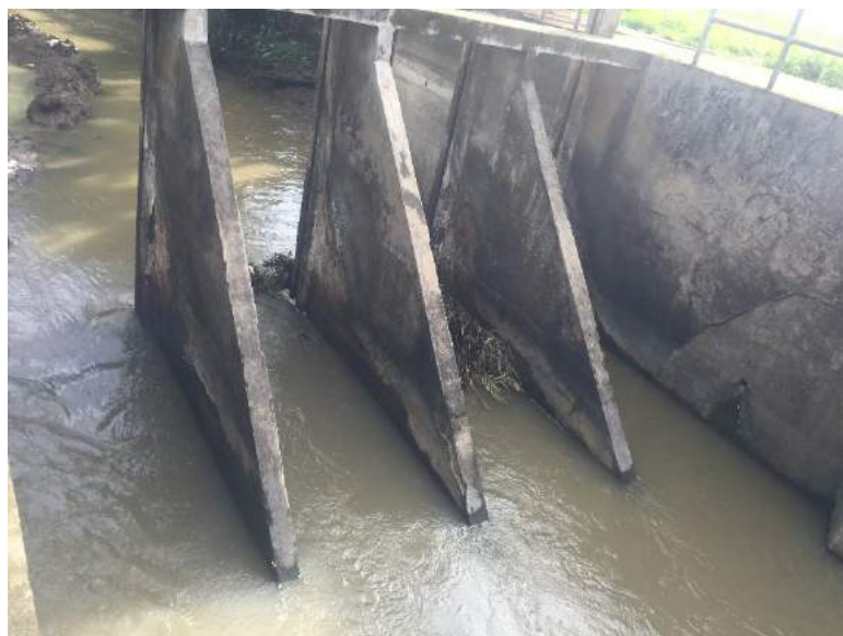
Figure 1B- 17. The buttress dam of Sta. Elena CIS. The IAs use wooden planks since no steel gates were installed
