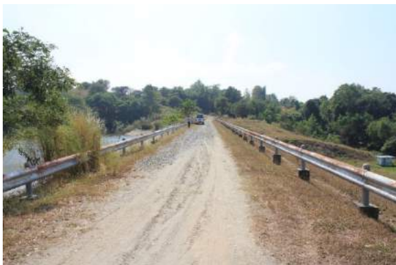
Figure 1A-44. The road atop the dam crest Source: Author’s capture
