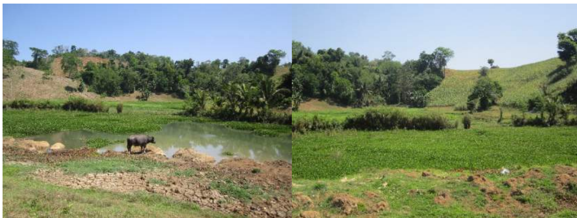
Figure 1A-97. The impounding reservoir filled with water lilies indicating heavy siltation
