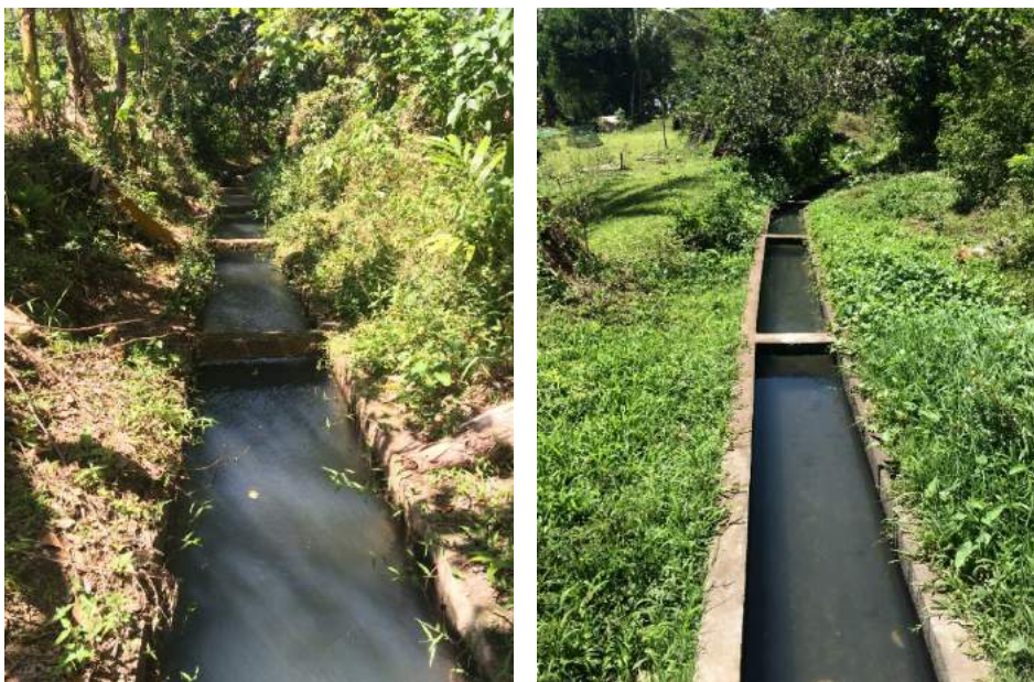
Figure 1A-67. Left: Upstream portion; Right: downstream portion of the rectangular main canal
