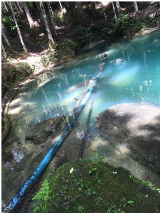
Figure 1B- 7. The three pipes also tapping water from the spring to provide water for the barangay (6"), ram pump for the High School (3"), and a private service area (3")
