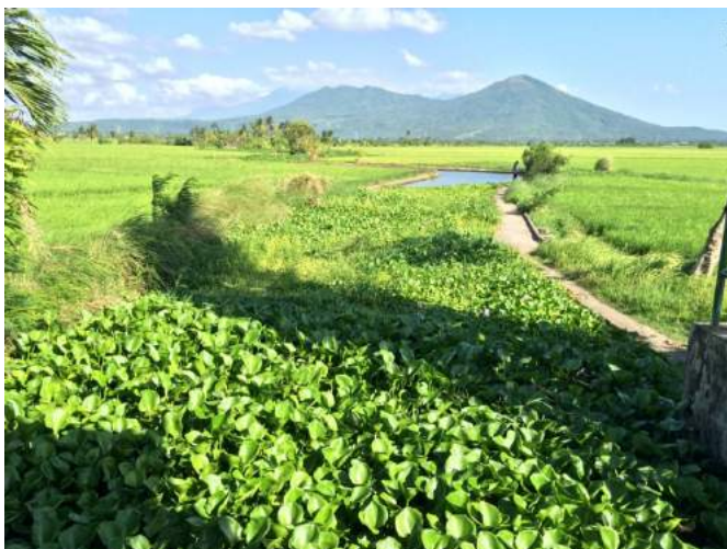
Figure 1A-107. Downstream portion of the dam that is full of water lilies
