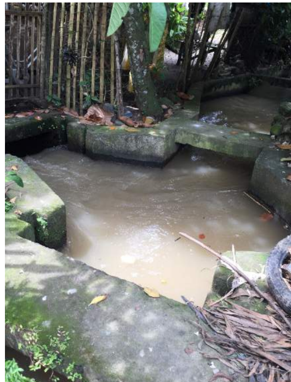
Figure 1C-20. The main canal and division box to divide flow from to different zones
