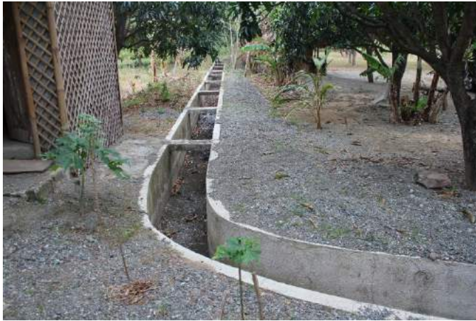
Figure 1A-27. The concrete-lined rectangular main canal
