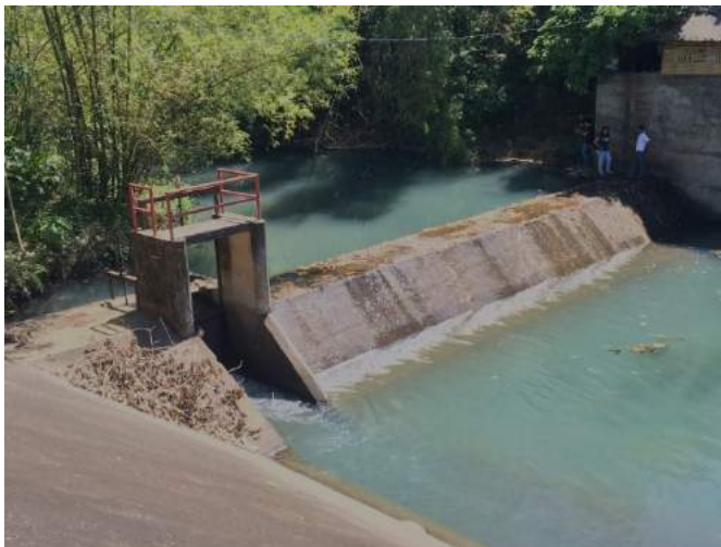
Figure 1A-66. Maybatang Dam
