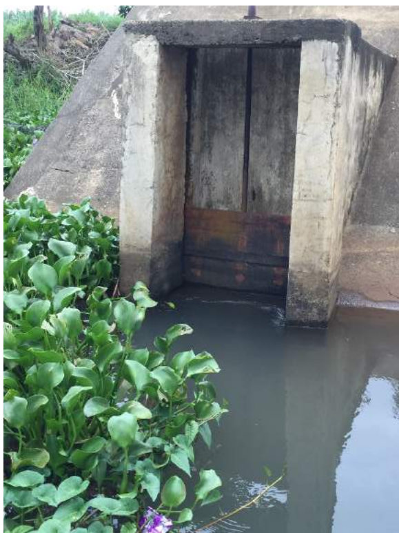
Figure 1C-39. Left main canal intake with 1 m width
