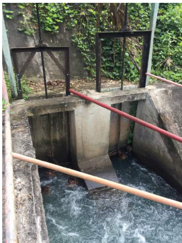
Figure 1C-11. The intake gates with the silt control structure funded by the IA
