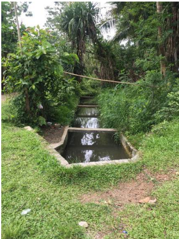
Figure 1B-2. The main canal of the Gabayan CIS Source: Author's capture
