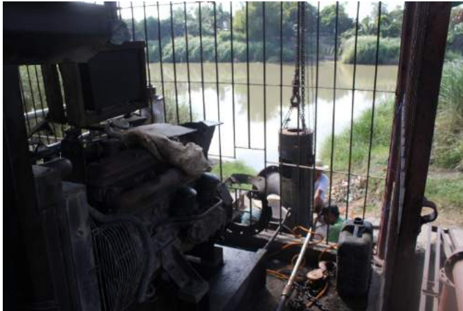
Figure 1A-2. One of 2 Iveco diesel engines for the mixed flow pumps; at the background is the Pampanga River where the PIS derive its waters
