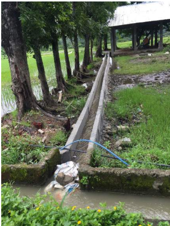
Figure 1B- 26. The newly built lateral canal of the system
