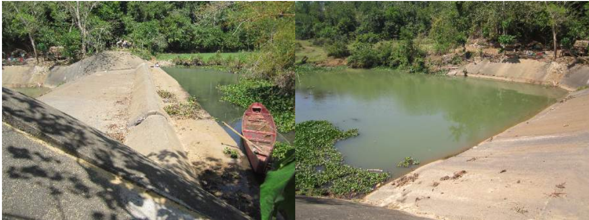
Figure 1A-98. The impounding dam upstream (left) showing crest height increased by a few feet where the overflow water goes downstream (right) to the brush dam
