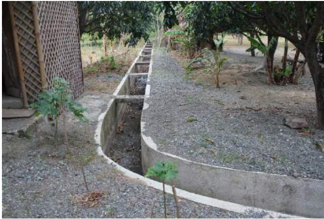
Figure 1A-27. The concrete-lined rectangular main canal
