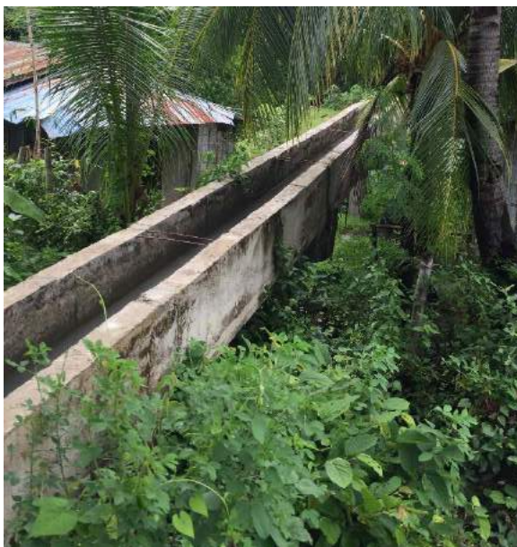
Figure 1B- 27. Elevated flume of Siwaragan CIS
