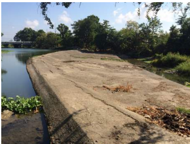
Figure 1A-58. The Zanjanera Bangsirit CIS dam
