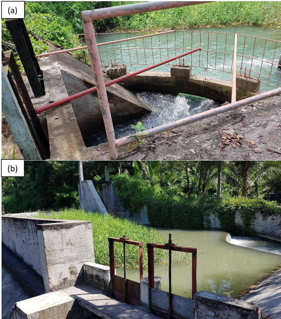
Figure 27. Silt control device in (a) Del Carmen CIS (Marbel River, N. Cotabato) and (b) LMT CIS (Taplan River, S. Cotabato).
