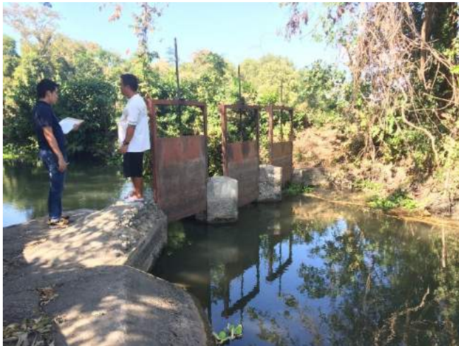
Figure 1A-59. The intake structure of the dam
