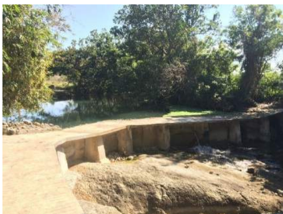
Figure 1A-63. The simple concrete dam of the Der-Ap Saoit CIS
