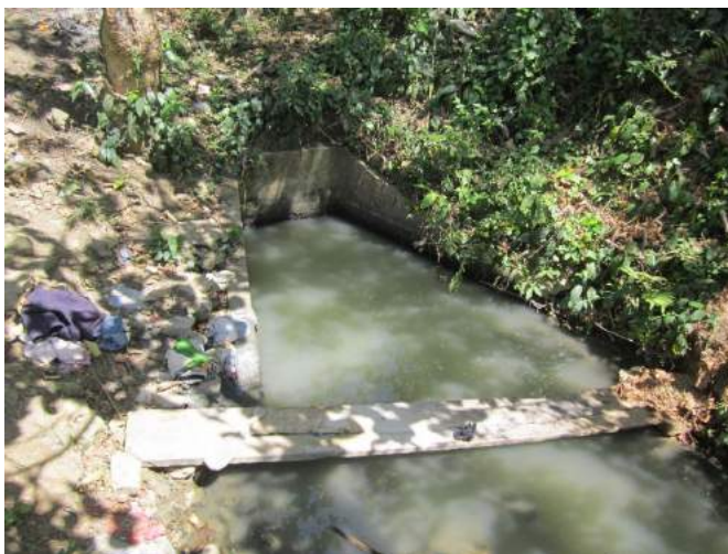
Figure 1A-100. The outlet from the intake gate leading to the trapezoidal main canal
