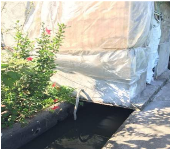
Figure A1-109. A drainage outlet of a house alongside of the main canal
