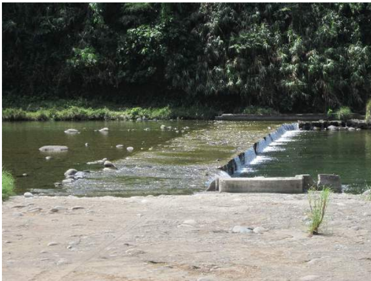
Figure 1A-87. The old dam (top) and the repaired part (bottom); the old intake can be seen in between the two
