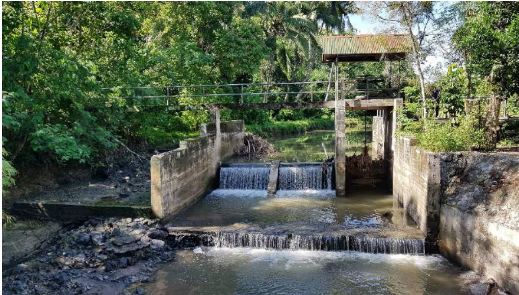
Figure 1C-25. The dam of Mani CIS with a sluice gate of 2 m width Source: Author's capture
