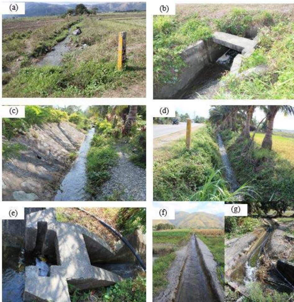
Figure 1A-35. (a) An unlined secondary canal; (b) a concrete check gate and inlet to a road crossing; (c) a lateral at the side of the highway which has a riprap side wall; (d) an unlined lateral at the side of the highway; (e) a concrete check gate in a lateral; (f) a concrete-lined lateral; (g) domestic water supply flexible pipes along a lined lateral
