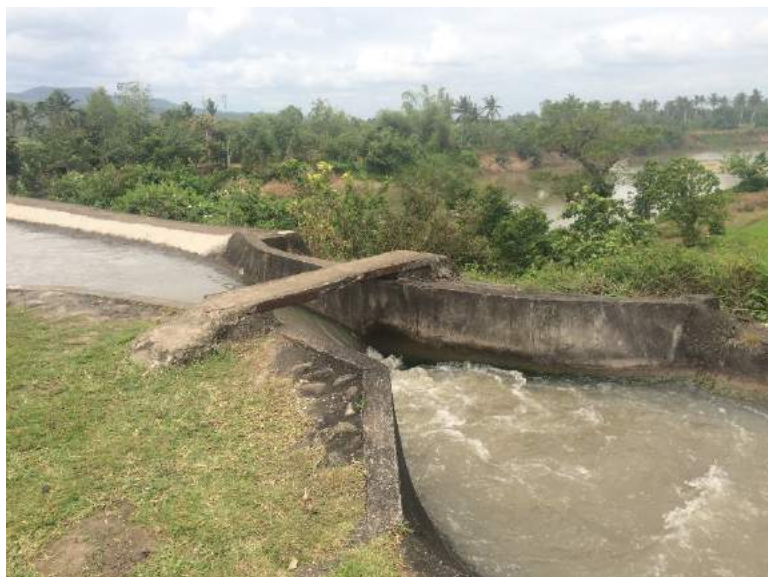
Figure 1A-70. Parshall flume in the upstream part of the main canal
