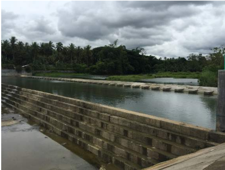
Figure 1B- 13. The diversion dam of Tagbawto CIS with a width of 100 m Source: Author's capture
