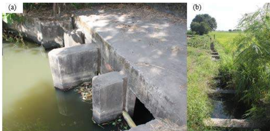
Figure 1A-20. (a) The check gate which the IA refers to as “Dam 2” is used to increase the head at the main canal for distribution to secondary laterals; (b) one of the laterals (concrete-lined) served by the check gate
