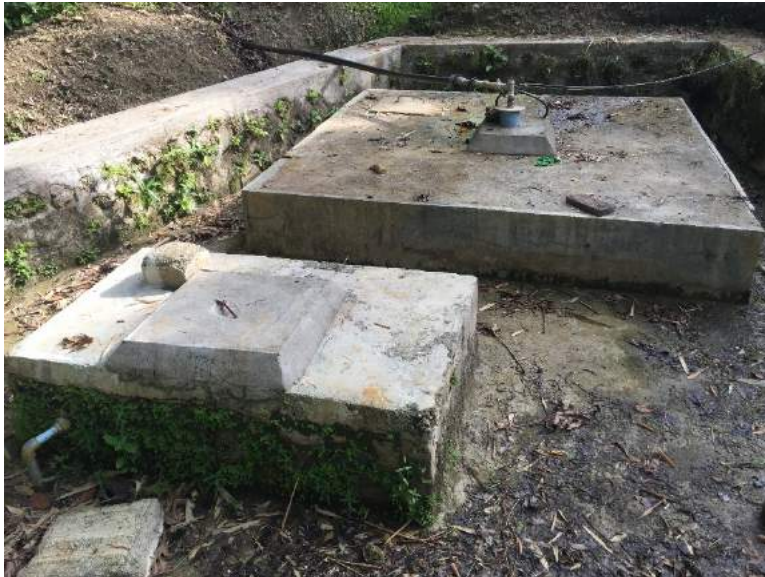
Figure 1B-4. The well source of Loboc Groundwater IP showing the two reservoirs
