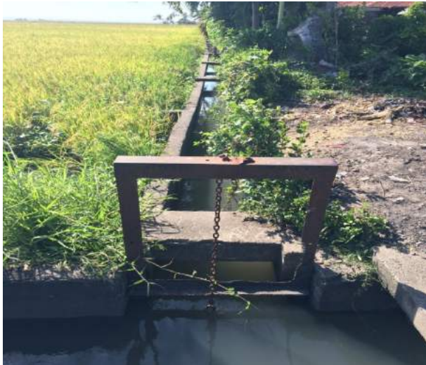
Figure 1A-108. Lateral canal without gate and lock
