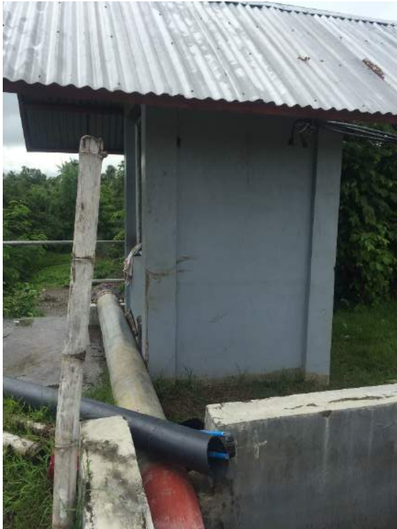
Figure 1B- 22. The 10” pipe (a) connected to the original pump and the 6” pipe (b) connected to the alternative pump
