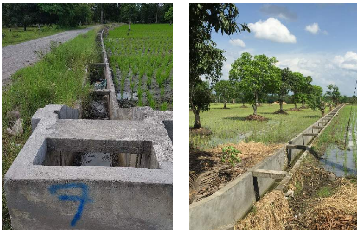
Figure 1C-9. Lined main canal of the Butilon CIS
