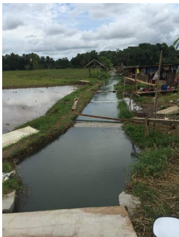
Figure 1B- 12. Ongoing canal construction with width of 2 m and depth of 1.25 m
