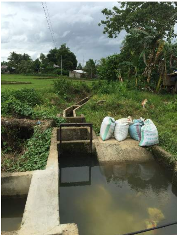
Figure 1B- 33. Lateral canal A and division box of the system
