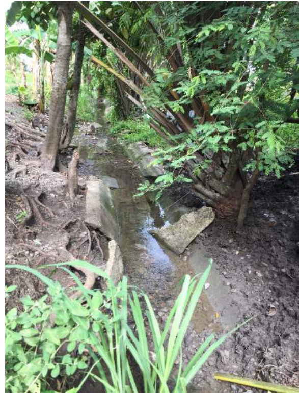
Figure 1C-6. The unlined and broken portions of the main canal
