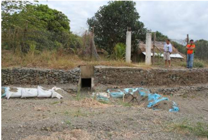
Figure 1A-24. The intake gate upstream of the dam use wooden slabs as gates; the gabions serving as side embankments of the dam are damaged; sand bags used to divert the depleting water last cropping are also shown
