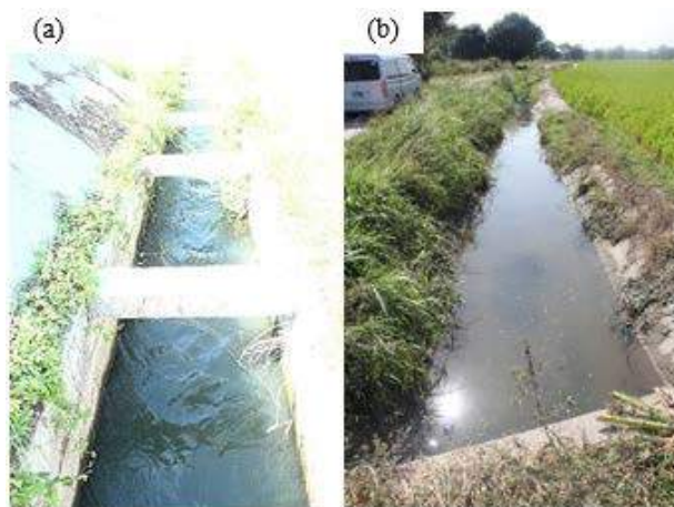
Figure 1A-18. (a) Rectangular portion of the main canal parallel the mega-dike immediately downstream of the dam; (b) trapezoidal portion of the main canal
