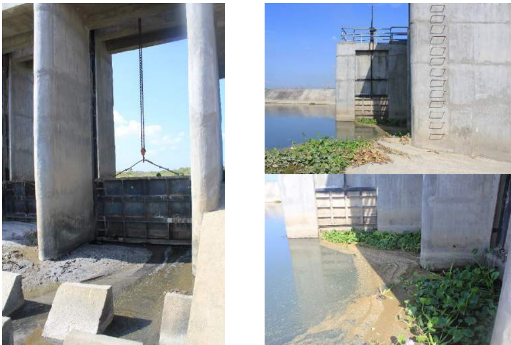
Figure 1A-17. Clockwise from left: (a) the two sluice gates showing some siltation and leakage, also shown are the baffle blocks; (b) The intake structure was designed to be near the middle of the river, the intake gates are still functional; (c) the approach to the sluice gates and intake gates are heavily silted
