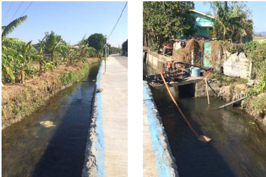
Figure 1A-62. Lateral canals: Left – grasses are growing at the channel bottom; Right – a low-lift pump (LLP) extracting water from the canal (according to the farmer interviewed, the owner of this pump is not a member of the IA).
