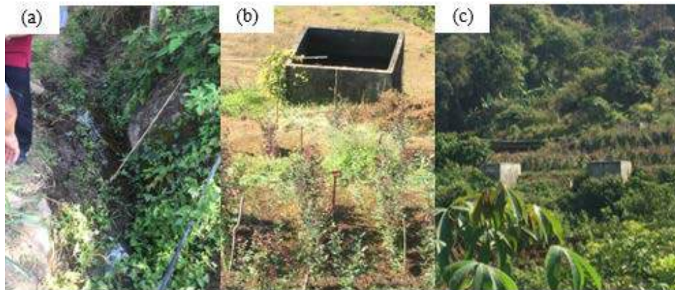
Figure 1A-80. (a) Unlined main canal used to irrigate rice (b); (c) some of the concrete tanks
