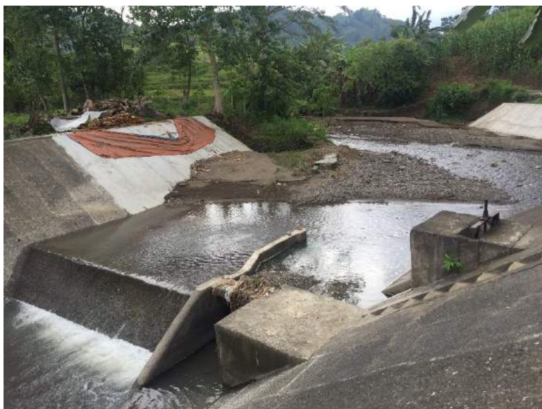
Figure 1C-45. Dam 2 of the system wherein the sand also enters the intake gate
