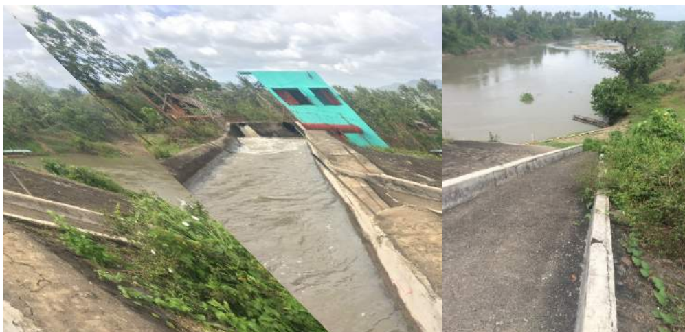
Figure 1A-69. The spillway leading excess water back to the Bicol River
