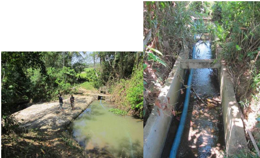
Figure 1A-101. The brush dam now made of concrete and the rectangular lined canal constructed by the IA; water is pumped to the canal due to low flow
