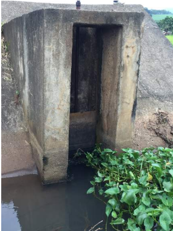
Figure 1C-38. Right main canal intake with 0.5 m width
