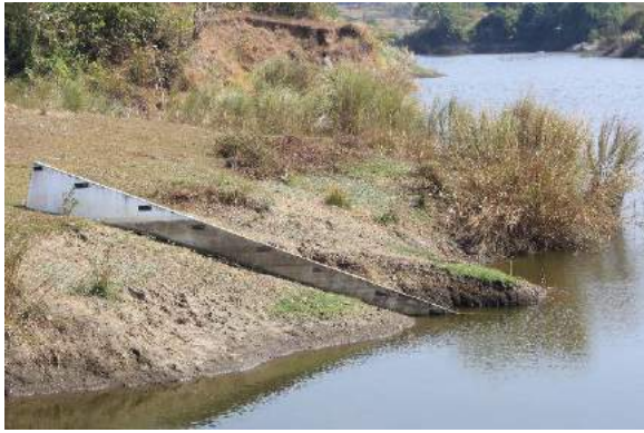
Figure 1A-46. The water level gage meter made of concrete reservoir of the San Angel SRIP; also shown are the rocks lining the slopes of the upstream face of the dam
