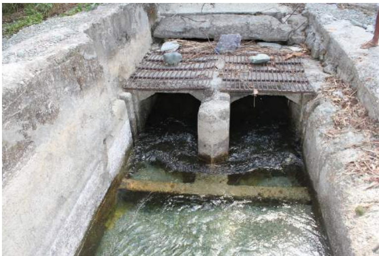
Figure 1A-30. The intake structure leading to the underground tunnel into the main canal
