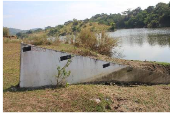
Figure 1A-46. The water level gage meter made of concrete reservoir of the San Angel SRIP; also shown are the rocks lining the slopes of the upstream face of the dam
