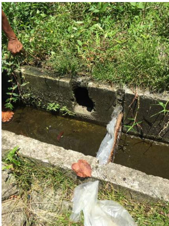
Figure 1C-31. Simple hole turnout and improvised gate
