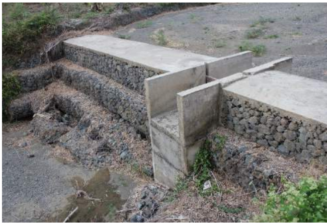
Figure 1A-22. The Cordero CIS dam along Arimal creek is made up of gabions and plastered with cement at the crest; shown at the left side are the damaged gabions where water seeped underneath the dam
