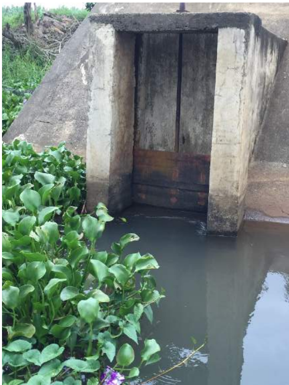
Figure 1C-39. Left main canal intake with 1 m width
