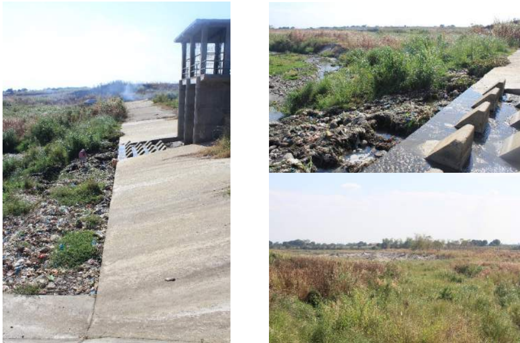
Figure 1A-16. Clockwise from left: (a) scouring at the downstream apron, the sluice gates and intake structures are seen at the middle of the dam; (b) the gabions are damaged and accumulating garbage; (c) the quarry operations just downstream of the dam location
