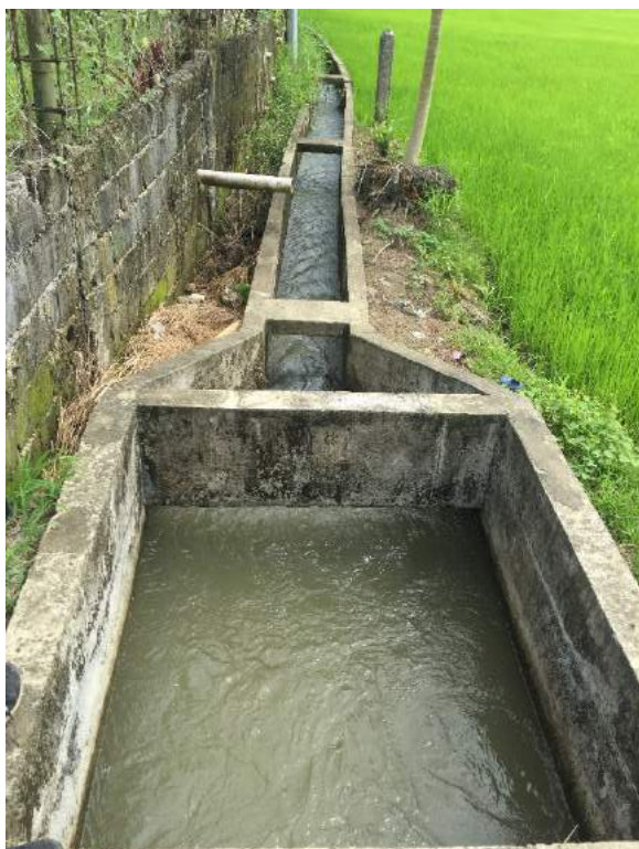
Figure 1B- 36. The main canal of the system as the canal emerged from an inverted siphon across a road
