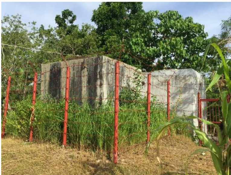
Figure 1B-5. The main (2m x 2m) and additional (2.5m x 2.5m) reservoirs of the system
