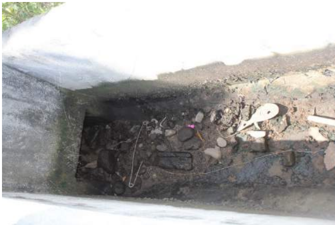
Figure 1A-11. Siltation and garbage observed from the portion of the main canal near the pump
