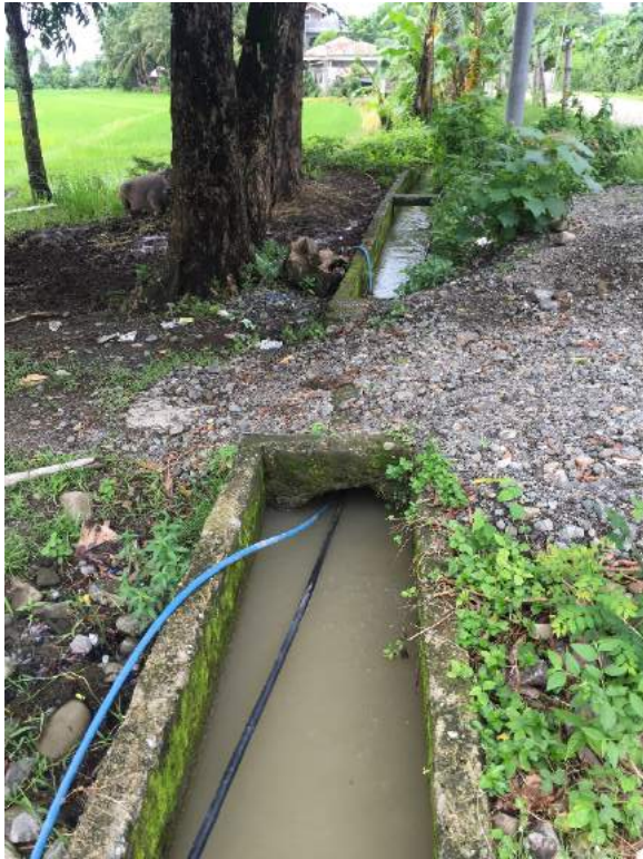
Figure 1B- 25. Main canal of Tumagboc CIS with width of 60 cm and depth of 60 cm
