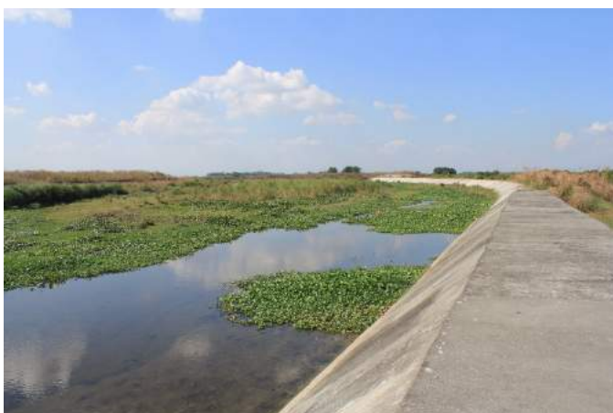
Figure 1A-15. The concrete embankment at the approach to the dam, again showing heavy siltation
