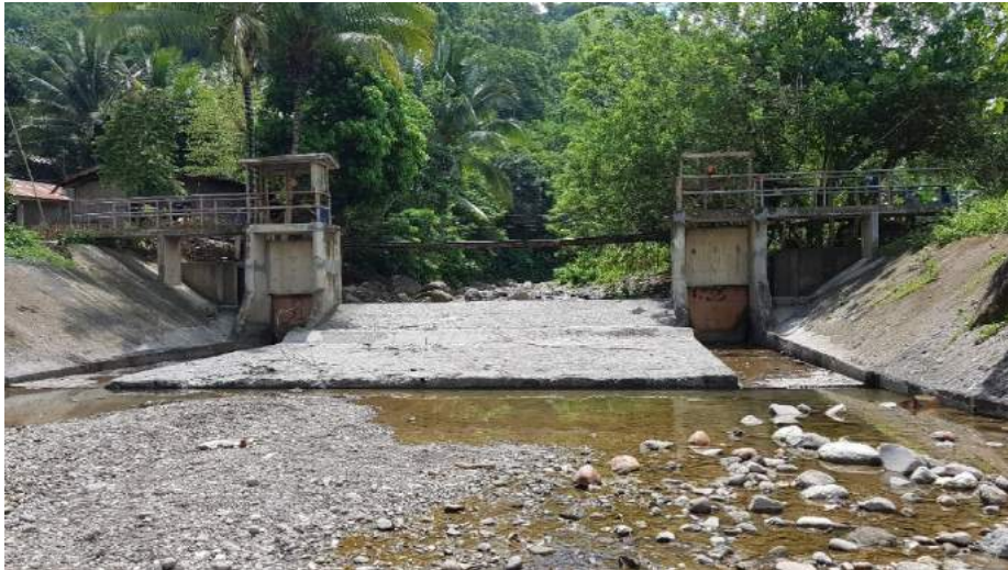
Figure 1C-32. The dam of Delapa CIS
