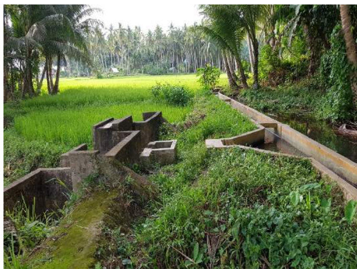
Figure 1B- 10. The original dam constructed in 1960 downstream of the new site. The main canal of the new dam is seen on the right side
