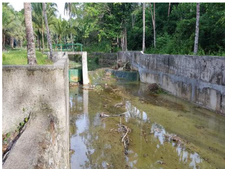
Figure 1B- 9. The new dam of the Maljo CIS constructed in 2012. It is a run-of-the-river type dam with a duckbill crest
