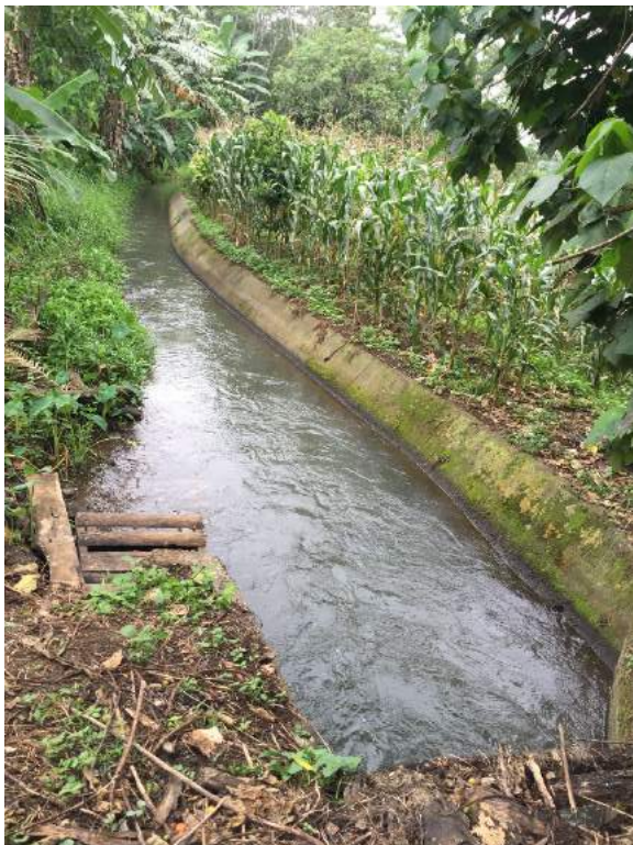
Figure 1C-41. Left main canal of the CIS Source: Author's capture
