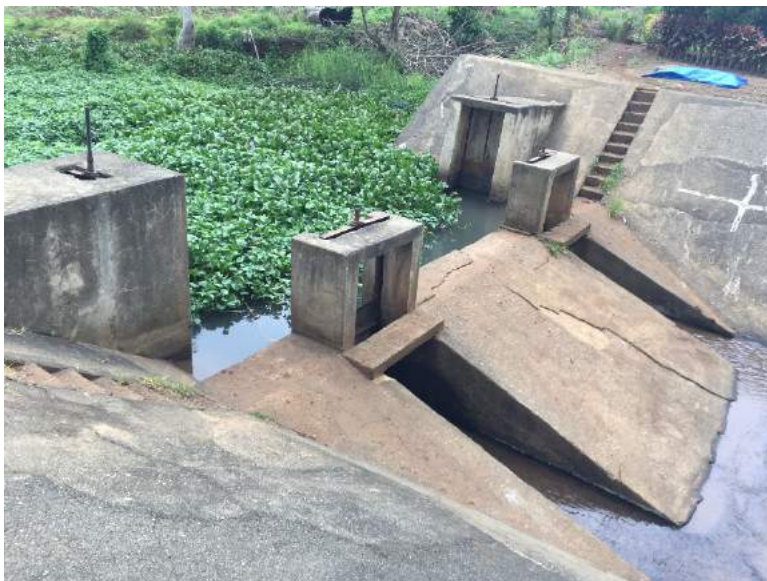
Figure 1C-37. The dam of the system
