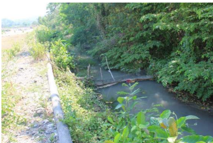
Figure 1A-113. The 2.5-m wide and 3-m deep concrete-lined main canal
