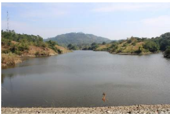
Figure 1A-45. The reservoir of the San Angel SRIP; also shown are the rocks lining the slopes of the upstream face of the dam Source: Author’s capture
