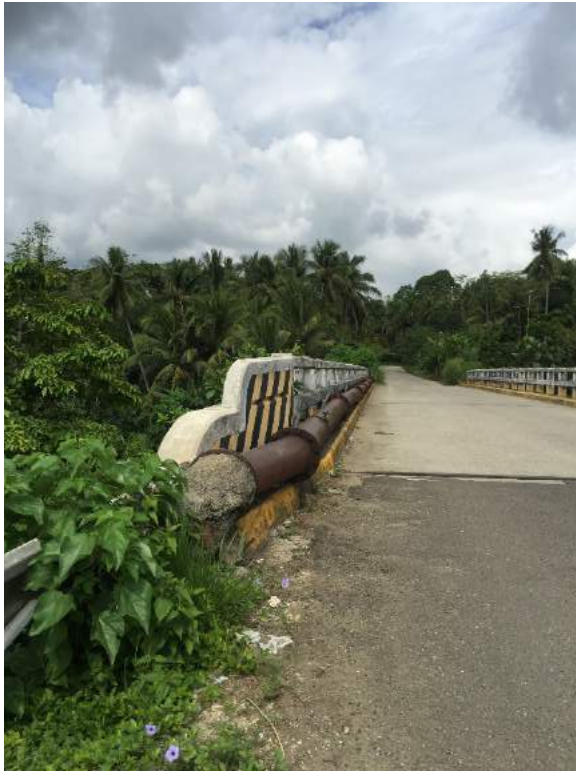
Figure 1B-3. Proposed alternative conveyance to the damaged inverted siphon of Gabayan CIS
