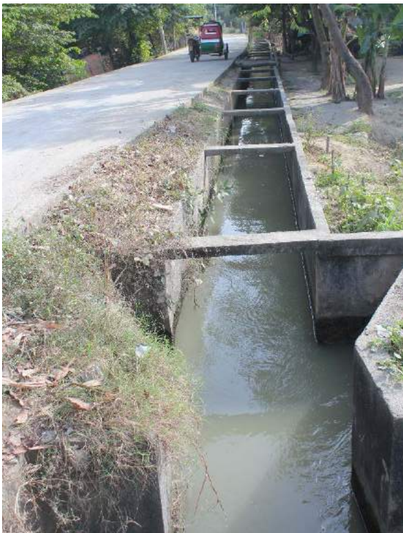
Figure 1A-6. The 1-m wide, 1-m deep concrete lined main canal of the Gulap PIS. The main canal and structures are well built since the IA said that they monitored the actual construction
