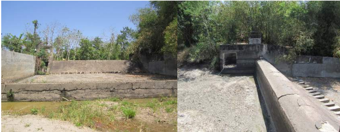
Figure 1A-94. The ogee dam exposed because there are no water on Pangul Creek during the visit; also shown is the bypass inlet used to divert water downstream during high flows
