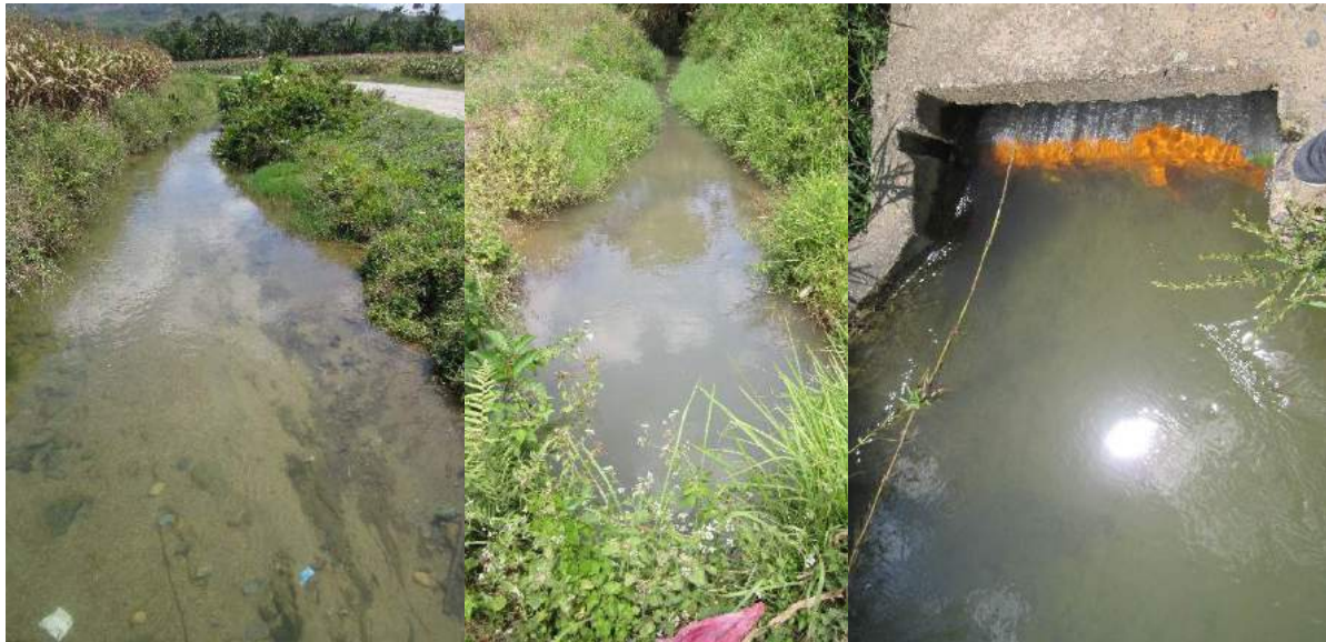
Figure 1A-91. The unlined main and lateral canal and one of the drop structure combined with siphon
