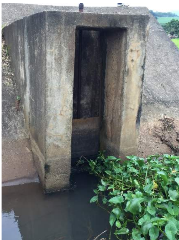
Figure 1C-38. Right main canal intake with 0.5 m width
