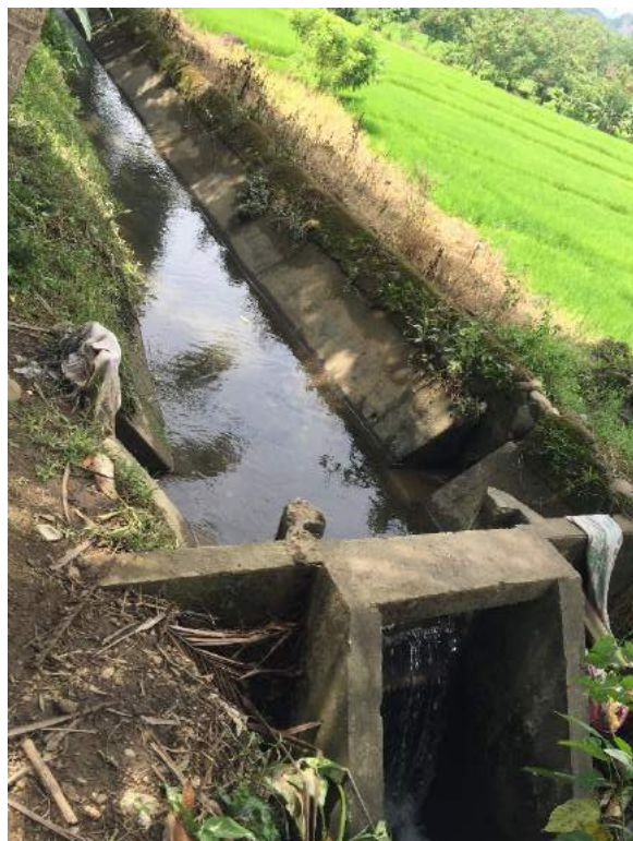
Figure 1C-35. Trapezoidal main canal of the system
