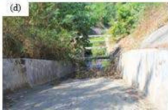
Figure 1A-47. (a) The entranceway to the concrete spillway; (b) the level spillway channel; (c) the hump along the spillway channel to increase storage capacity of the dam; (d) the spillway chute to channel excess water from the dam to a creek
