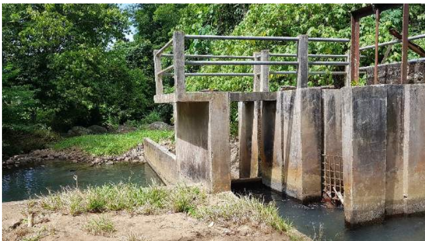
Figure 1C-2. Matanao Dam of Unifarm CIS
