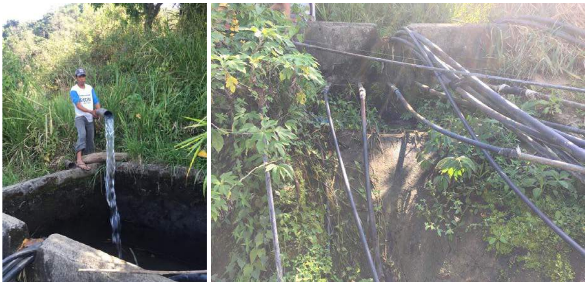
Figure 1A-79. The main tank showing flow of water from the source and the distribution pipes to the other tanks.
