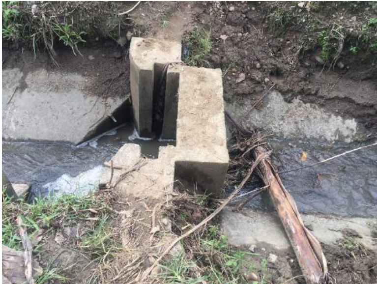
Figure 1C-48. Ejector for silts in main canal connected in Dam 2 Source: Author's capture
