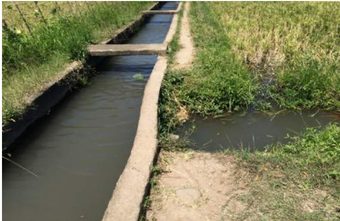
Figure 1A-103. The 1-m wide, 1-m deep concrete-lined main canal of Maria Pelaez CIS Source: Author's capture
