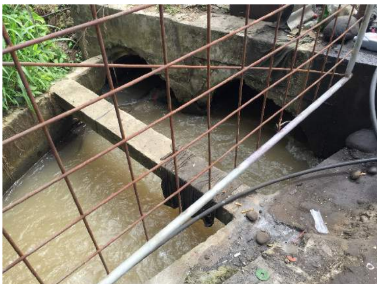
Figure 1C-21. Main canal of the system after the culvert road crossing
