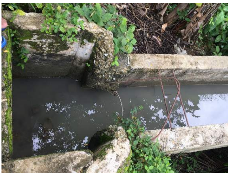
Figure 1B- 28. Connection of the main canal and the elevated flume showing the difference in width and height
