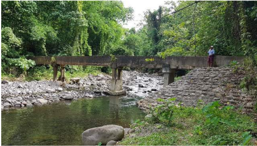
Figure 1C-3. Elevated flume from Matanao dam
