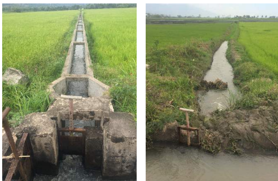
Figure 1A-71. Left: lined; Right: unlined farm ditches
