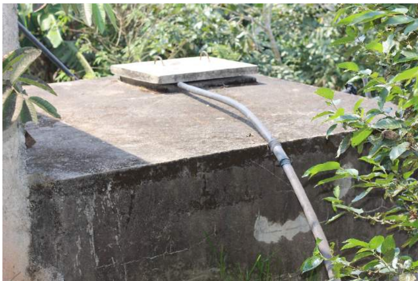
Figure 1A-84. One of the concrete storage tanks of the Taloy Sur CIS showing the entry point for tank cleaners
