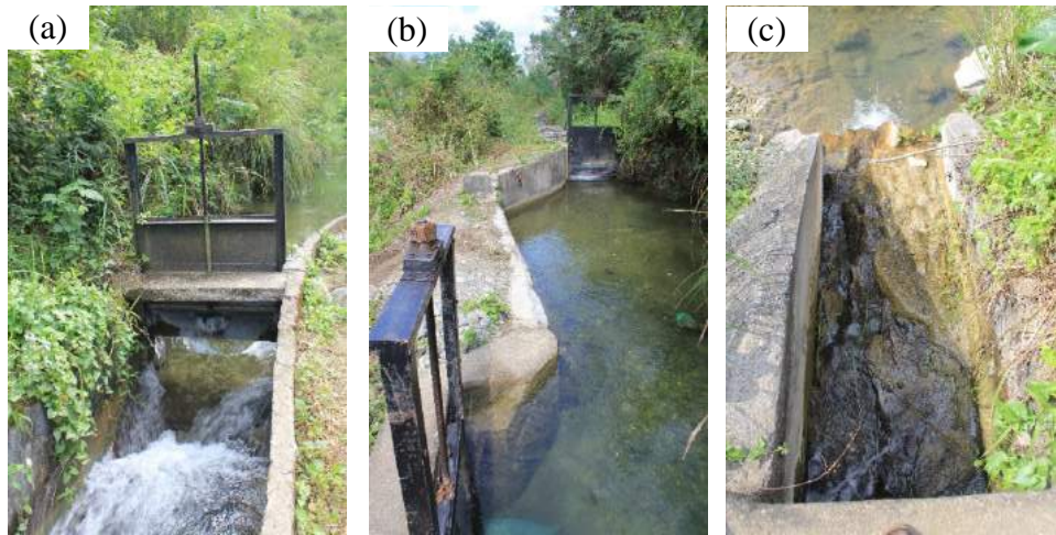
Figure 1A-40. (a) Check gate to control the flow to the main canal; (b) the gate at the top controls the flow to the main canal while the left gate controls return flow to the river; (c) guide chute for excess water reverted back to the river
