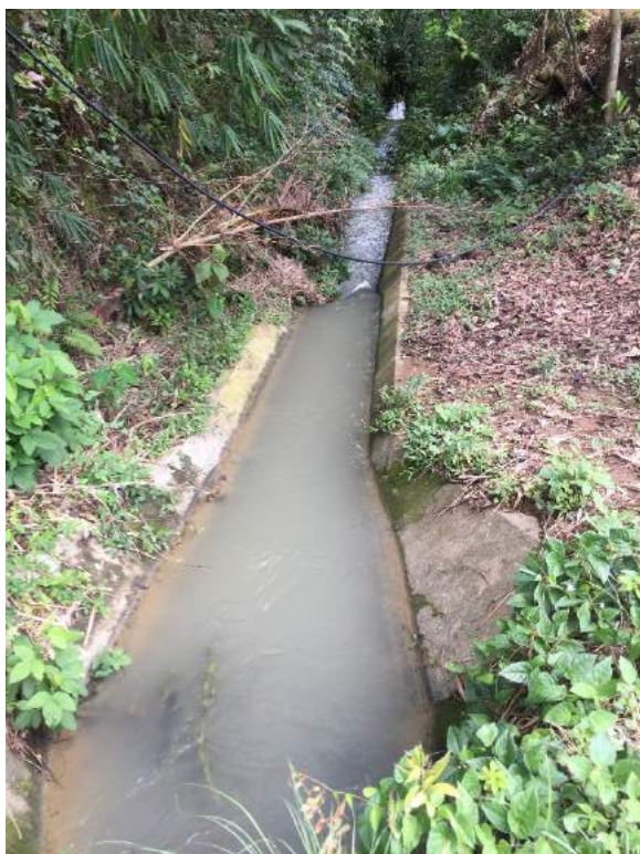
Figure 1C-47. Main canal connected to Dam 1
