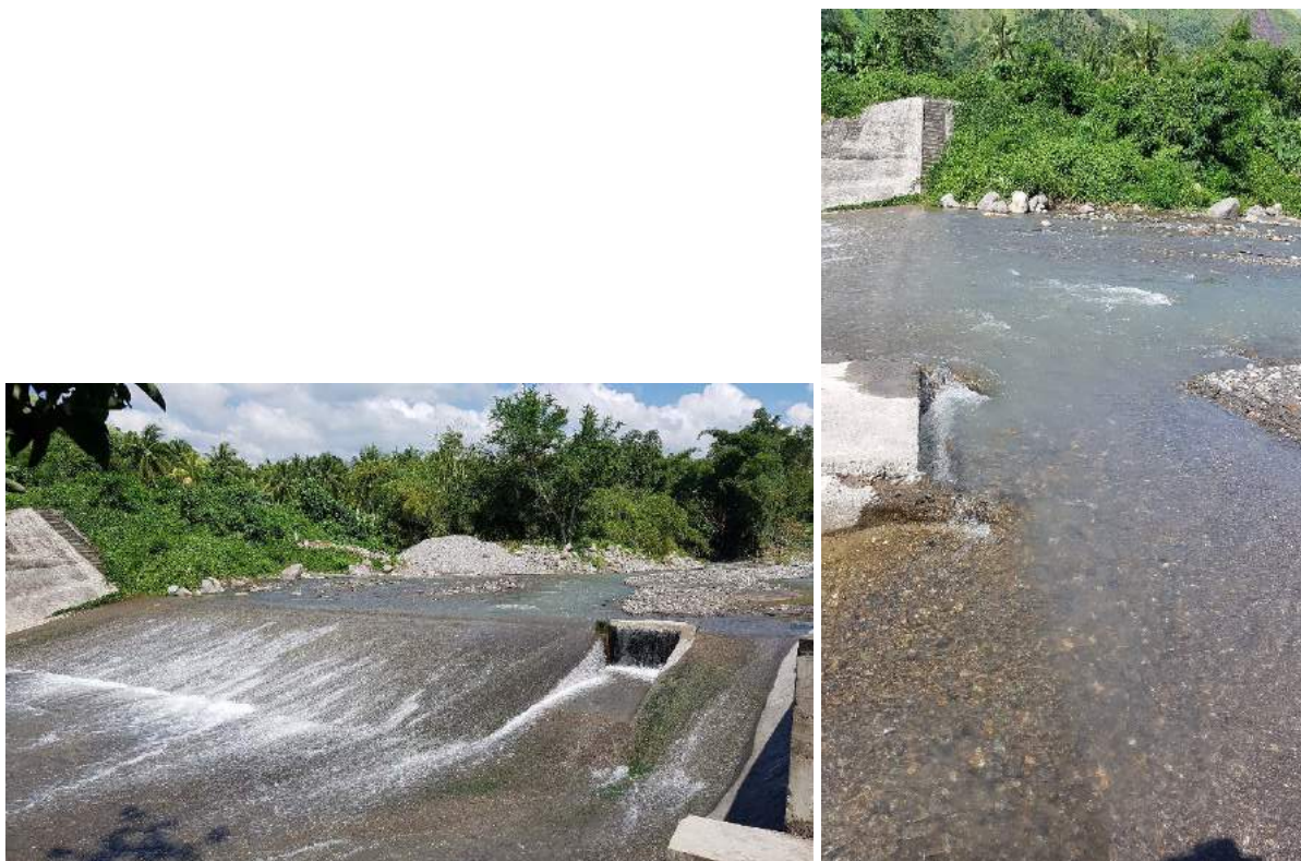
Figure 1C-22. The dam of LMT CIS filled with sediments
