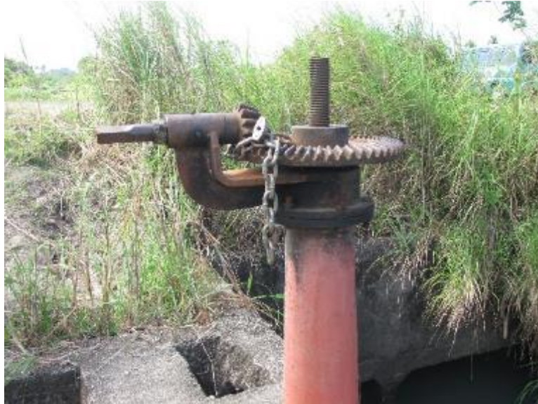
Photo 17. Check gate with padlocks in Libmanan-Cabusao PIS
