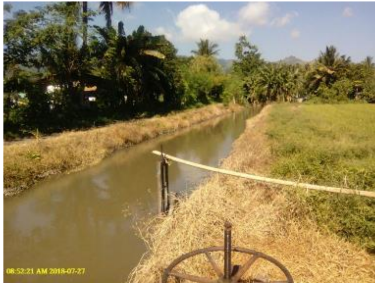
Photo 89. Silted section of Marbel #1 RIS.
