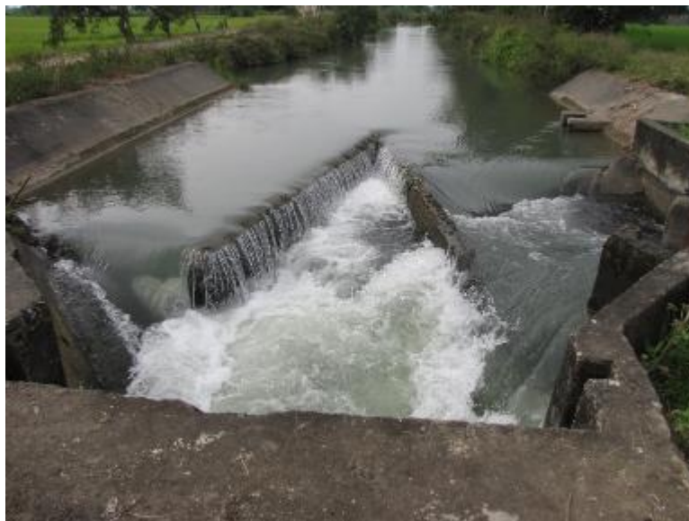
Photo 30. Control and division structures along Lateral B, Div.2, MARIIS. Take note of the damages and condition of the canal and structures.
