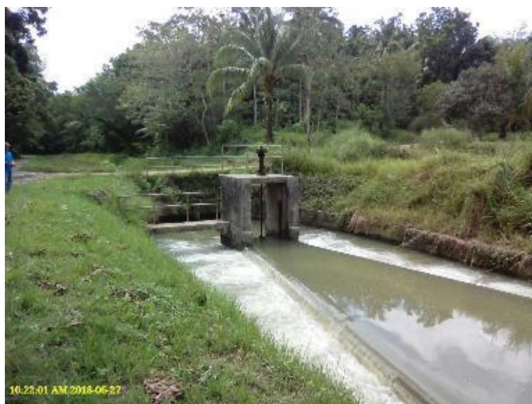
Photo 43. Duckbill weir near Lateral A, Malinao IS.
