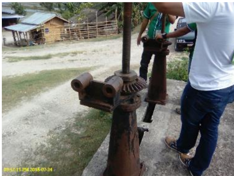
Photo 5. Missing gates in MalMar 2 RIS.
