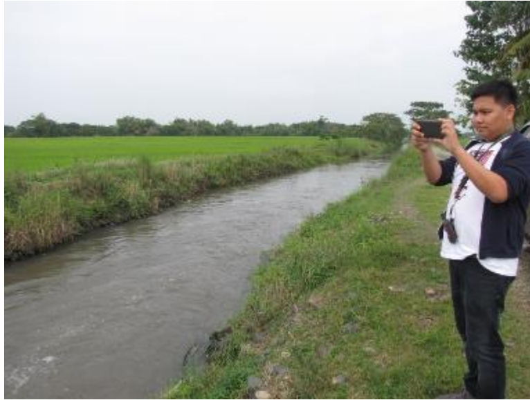
Photo 27. Unlined canal of Lateral B, Division II, MARIIS
