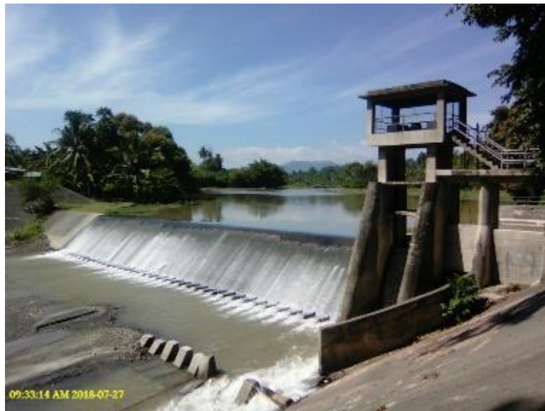
Photo 82. Diversion dam of Marbel #1 RIS.
